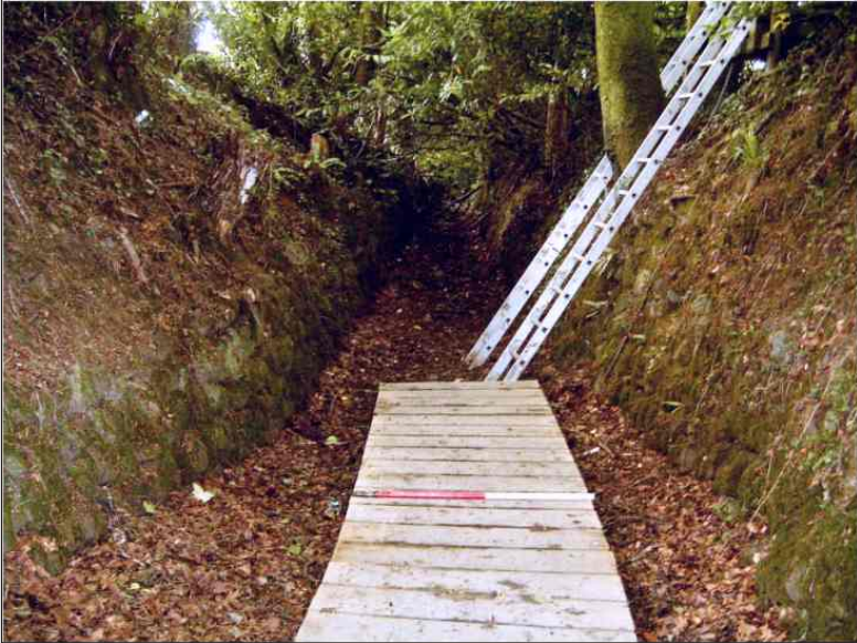
Plate 5: Town Leat at eastern boundary of development area, view from the east (scale 1m)
