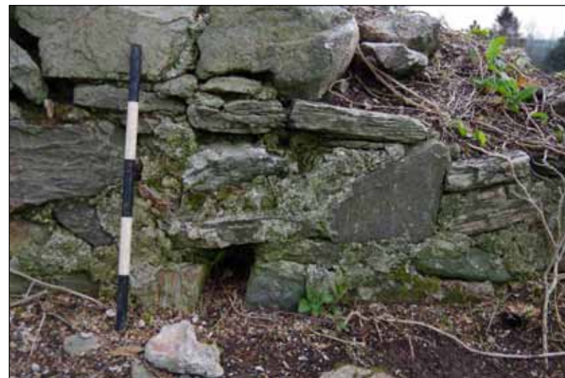
Plate 4: Zone 1, northeast wall interior, showing possible putlog hole and render, viewed from the west. 0.5m scale.
