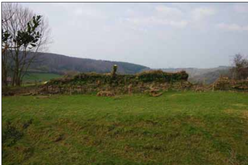
Plate 1: Zone 1, northeast wall exterior, south end, viewed from the east. 2m scale.
