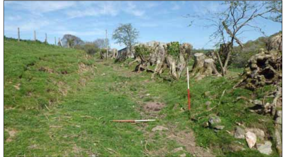
Plate 10: Zone 3, northeast end of green lane, viewed from the southwest. 1m and 1m scales.
