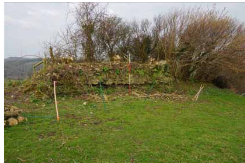
Plate 2: Zone 1, northeast wall exterior, north end, viewed from the southeast. 2m scale.
