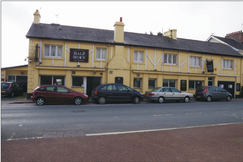
Plate 1: Northwest elevation of main range, looking southeast
