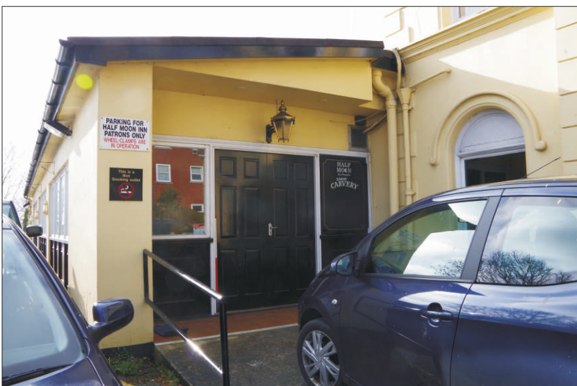
Plate 3: Northwest elevation of side extension, looking south (1m scale)
