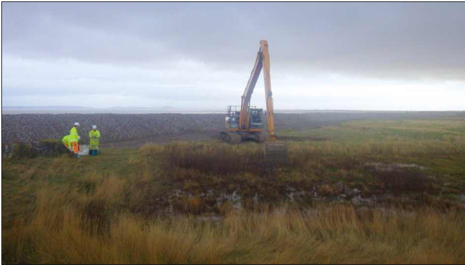
Plate 1: General working view of site looking northeast
