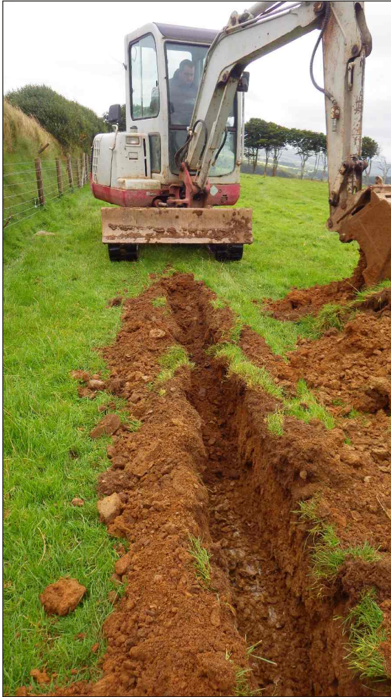
Plate 1: Trench 1, field 1, looking south along the eastern boundary
