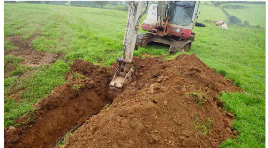
Plate 5: Trench 3, field 2, looking east
