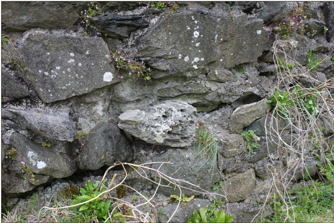
Plate 8: Stones 4 and 5, test fitting prior to consolidation, looking northeast
