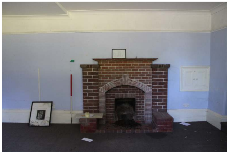
Plate 6: The fireplace and cupboard in room 1, looking east. (1m scale)
