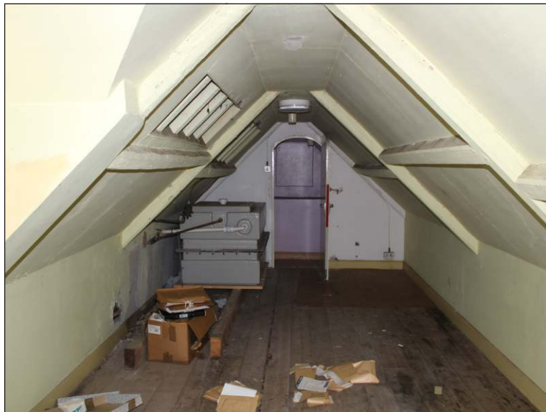
Plate 20: Room 12, general view showing roof construction, looking south. (1m scale)
