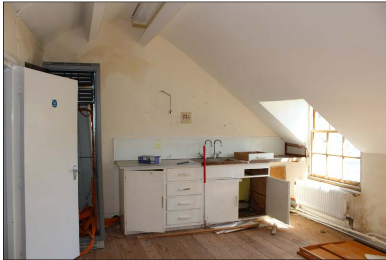
Plate 19: Room 10, general view showing purlins, looking east. (1m scale)
