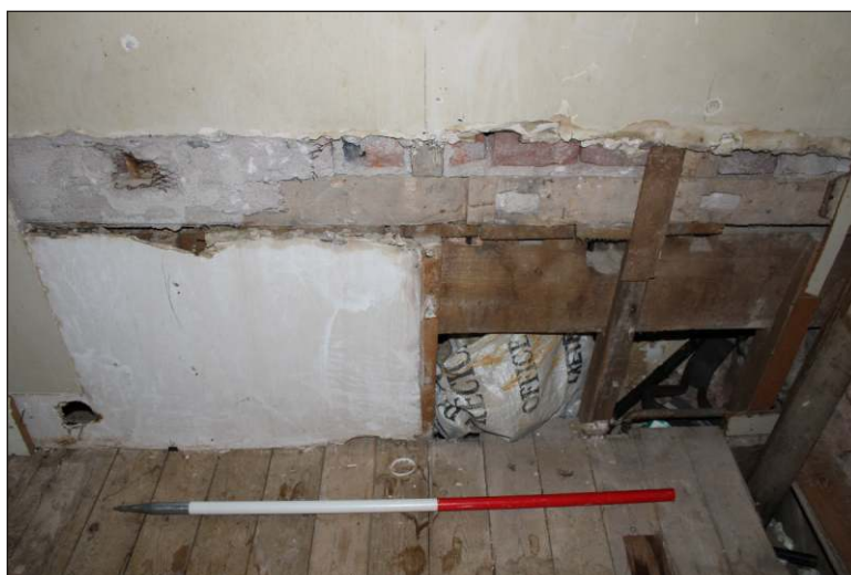
Plate 15: Room 7 showing construction of partition with kitchen, looking north. (1m scale)
