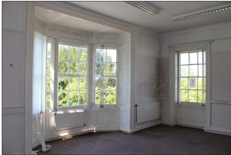
Plate 13: General view of room 5 showing the windows, looking northwest. (1m scale)
