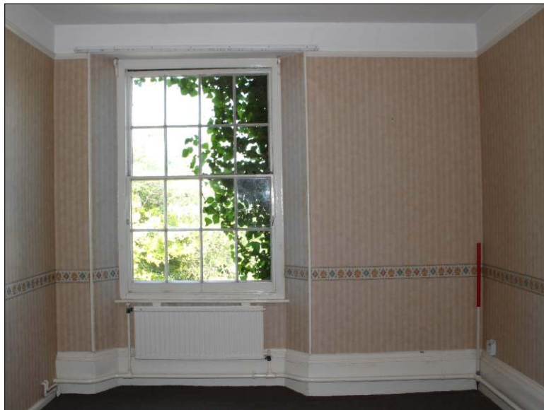
Plate 14: Room 6 showing walk-in window, looking north. (1m scale)
