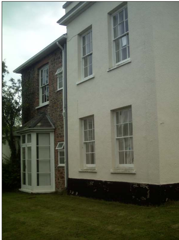
Plate 2: The north elevation showing the unrendered mid 19th-century extension, looking southeast
