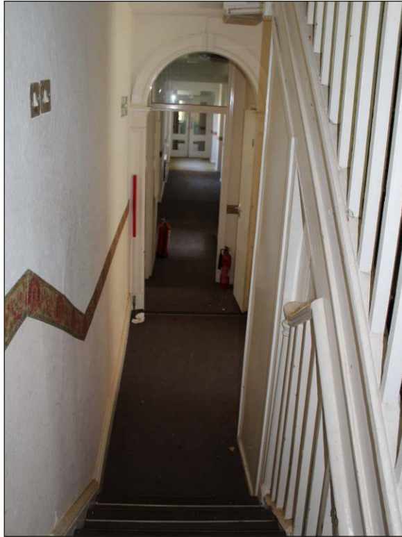
Plate 16: Corridor 4 and stairs to second floor, looking east. (1m scale)
