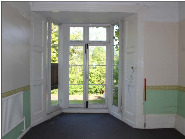
Plate 8: Room 3 showing the bay window, looking north. (1m scale)
