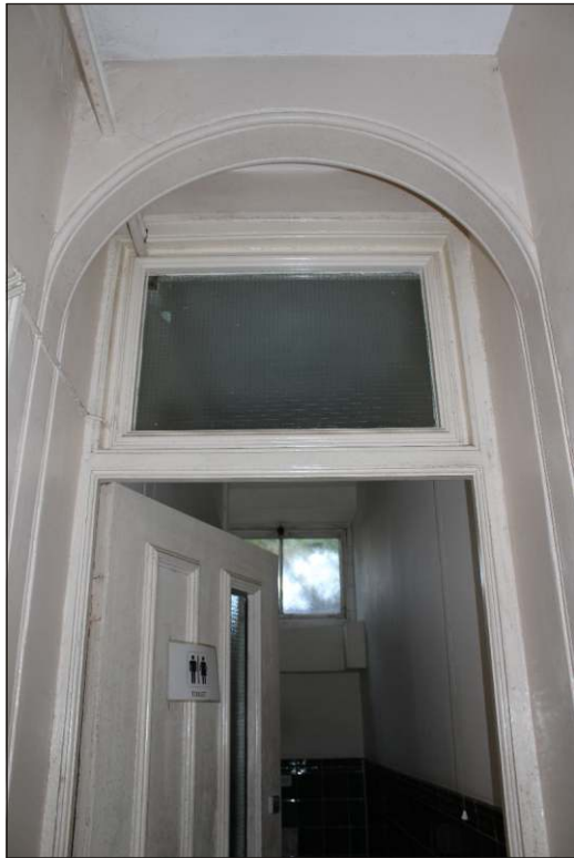
Plate 10: Arched opening in corridor to WC1, looking east
