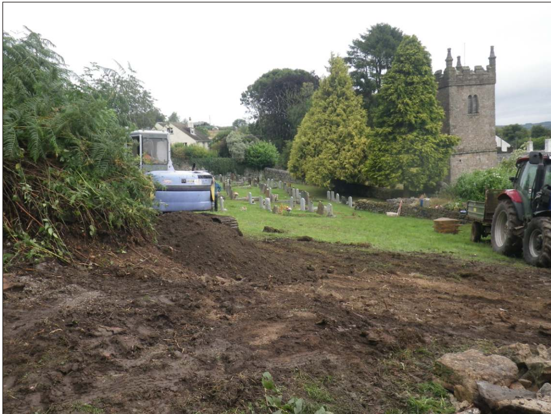
Plate 1: General view of site, looking north
