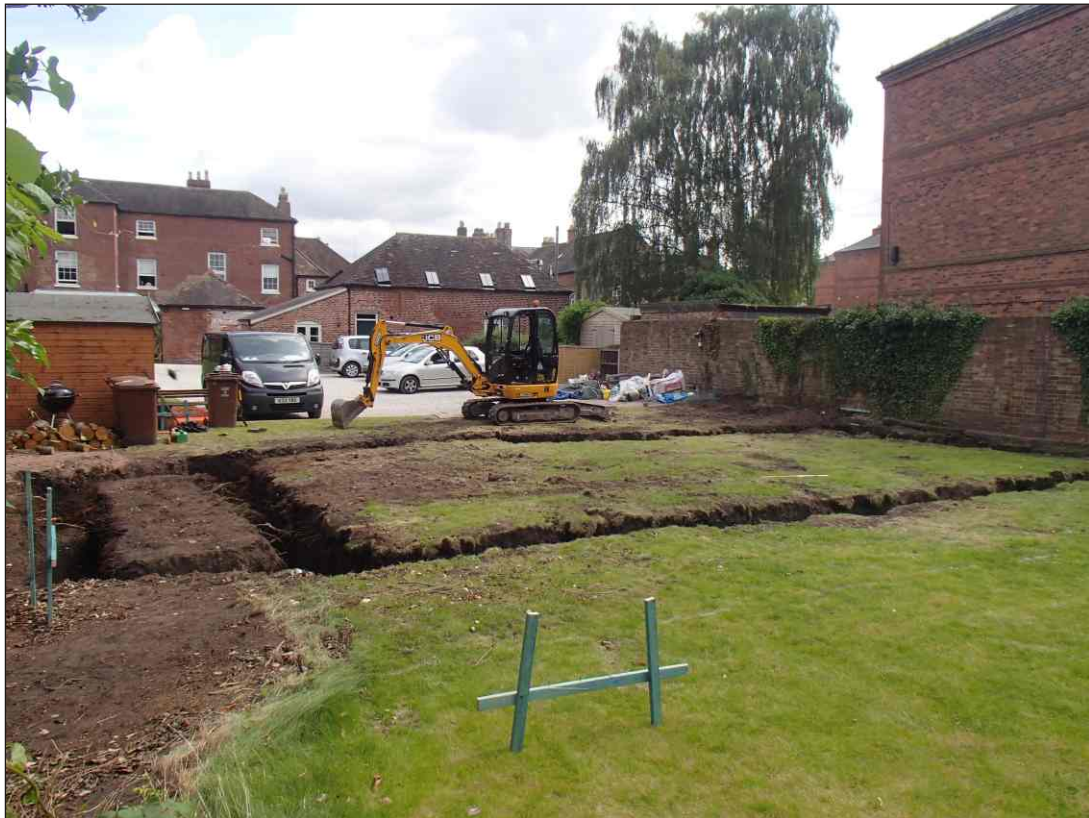
Plate 1: General view of site, view to the northeast. (Scale 1m)
