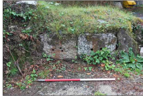
Plate 2: The track setts within the boundary, looking northwest. 1m scale
