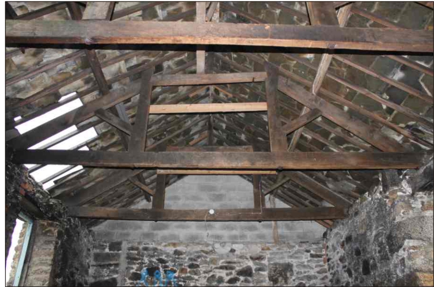
Plate 11: The roof structure, looking southeast
