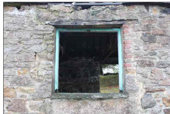
Plate 5: Detail of an inserted window in the northeast elevation, looking southwest
