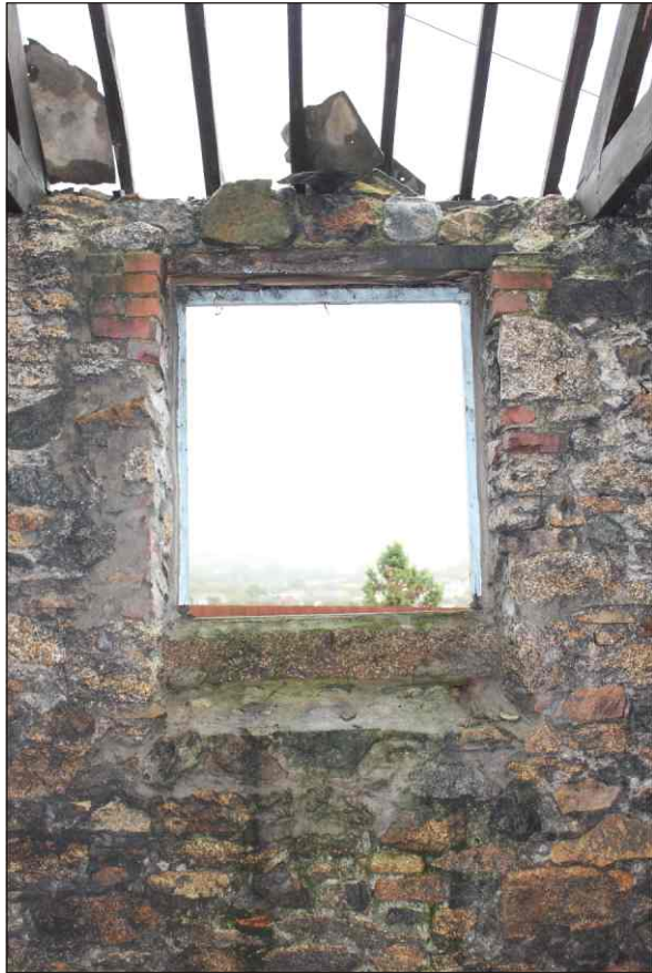
Plate 10: Detail of an inserted window in the northeast elevation, looking northeast
