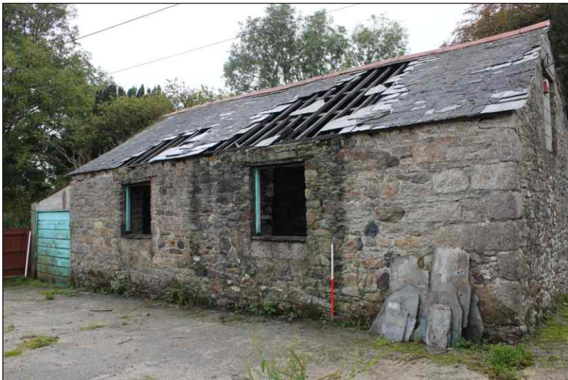
Plate 4: The northeast elevation, looking south. 1m scale
