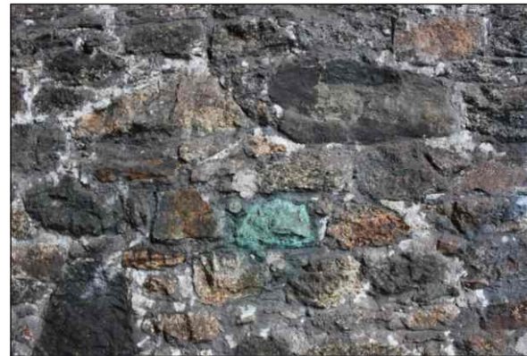
Plate 3: Masonry of the goods shed showing a copper-stained rock, looking southeast
