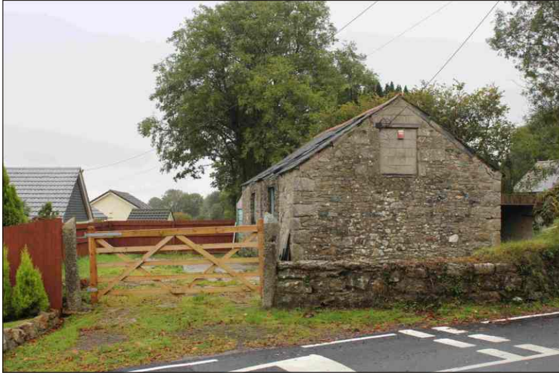
Plate 1: The goods shed showing its relationship to the line of the Liskeard & Caradon Railway to the left, looking southeast
