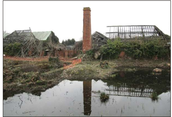
Plate 26: Building L1, complete southwest elevation and chimney, with northwest (left) and southeast (right) wings, from southwest
