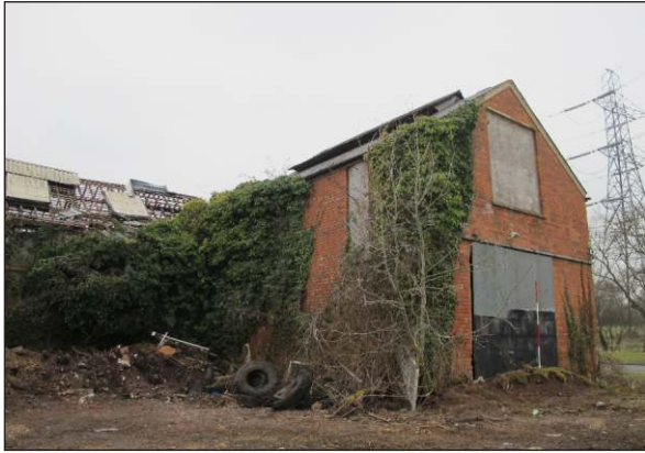
Plate 19: Building GR3 exterior, southeast and northeast elevations, from east. (2m scale)
