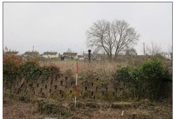
Plate 54: Round filter bed RF1 wall with voids and collecting channel in front, from northwest. (2m scale)
