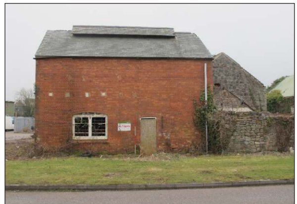
Plate 18: Building GR3 exterior, northwest elevation with GR4 on right, from northwest. (2m scale)
