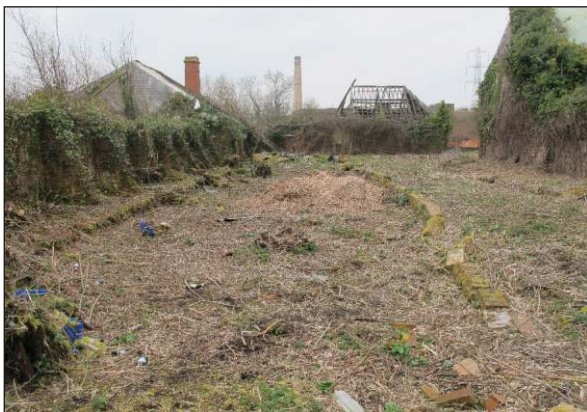
Plate 53: Filter bed B1 with low brick walls, from northeast. Buttressed filter tank BFT on left
