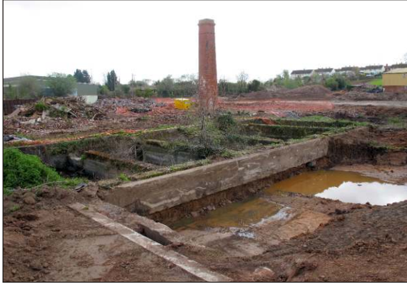
Plate 43: Five linked concrete tanks (T2), with filter bed B3 drained and cleared down to clay in foreground, from west
