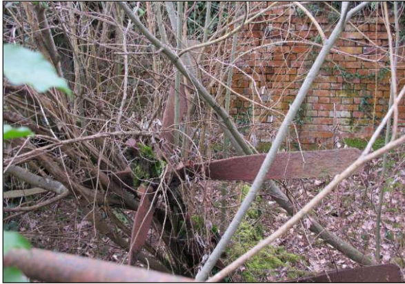
Plate 51: Buttressed Filter Tank (BFT). Twin iron 'paddles' inside chamber 5, from northeast
