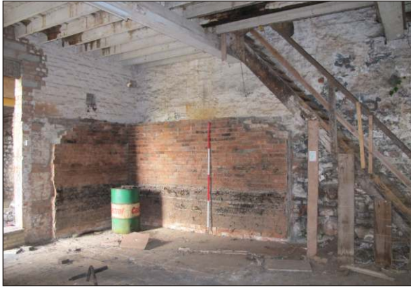
Plate 9: Building GR1 interior of Room A, with remains of tank 1 and stairs, from south. (2m scale)
