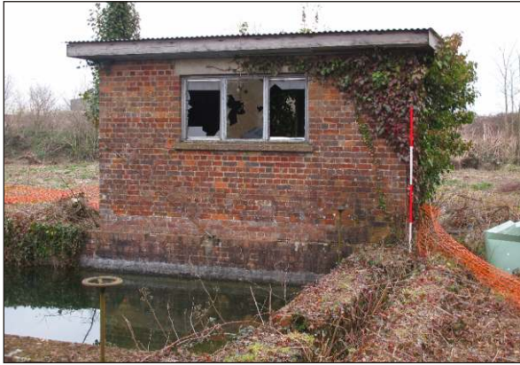
Plate 37: South pump house PH2 exterior, southwest elevation, from south-southwest. (2m scale)
