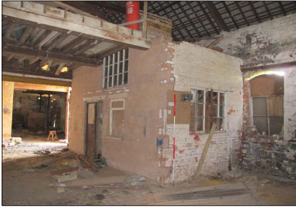
Plate 13: Building GR1 interior of Room B showing early wall and newer concrete block 'Office' wall, from north. (2m scale)
