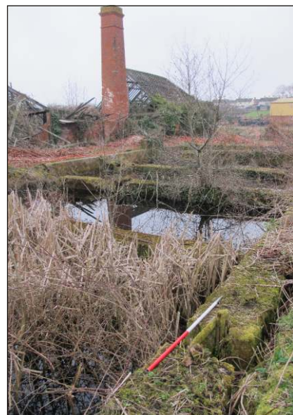
Plate 42: Five linked concrete tanks (T2) close to Building L1, with remains of wooden sluice from a channel in the foreground, from west-northwest. (1m scale)
