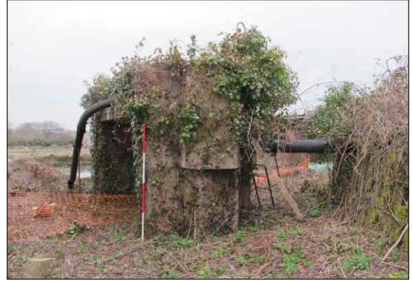
Plate 56: Concrete flow control feature RF2 associated with round filter bed, from south. (2m scale)
