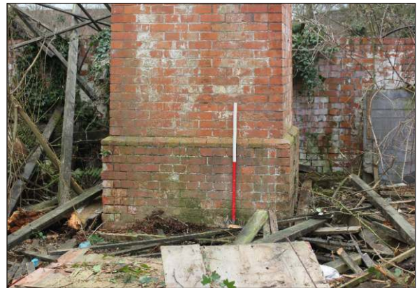
Plate 34: Chimney stack L2 base, from northeast (1m scale)
