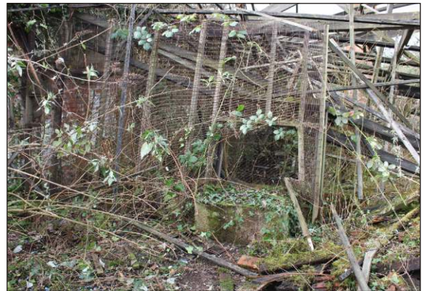
Plate 28: Building L1, interior of northeast wing with concrete base, collapsed metal screens and tank beyond, from east
