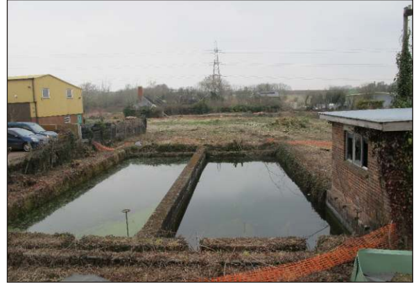
Plate 44: Twin tanks T4, channels and south pump house PH2, giving a good view over the site, from southeast
