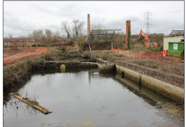
Plate 40: Main settling tank T1, general view with water partly drained, from northeast
