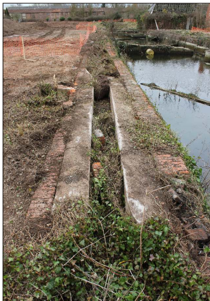
Plate 59: Channel C3 exposed on southeast side of main settling tank T1, from northeast. The associated chart flow recorder box F1 has been removed
