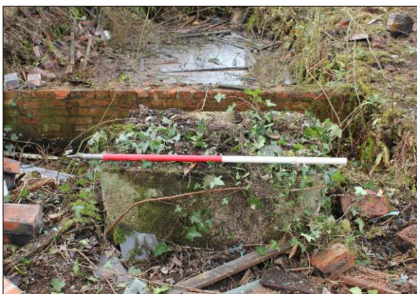
Plate 29: Building L1, interior of northeast wing after clearance, showing concrete base and tank, from northeast. (1m scale)
