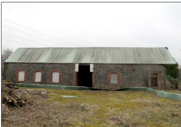
Plate 5: Building GR1, complete southwest elevation, from southwest. (2m scale)
