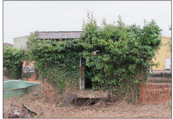
Plate 38: South pump house PH2 exterior, northeast elevation with overgrown door and steps, from northeast. (2m scale)
