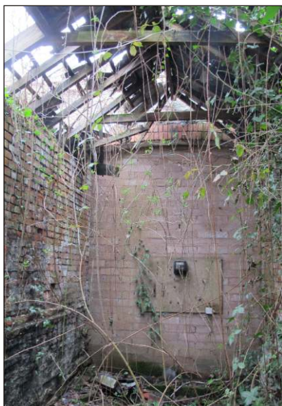
Plate 23: Building GR5, interior showing roof and blocked arch into GR2, from northeast
