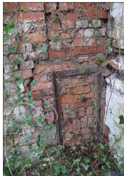
Plate 24: Building GR5, iron frame for draught regulating plate in northwest wall, from south-southeast
