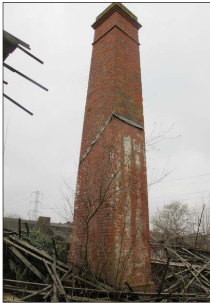
Plate 33: Chimney stack L2, from east
