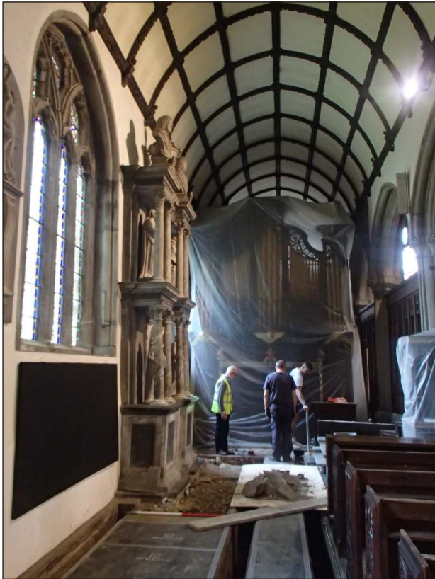
Plate 1: North aisle, works in progress, looking east
