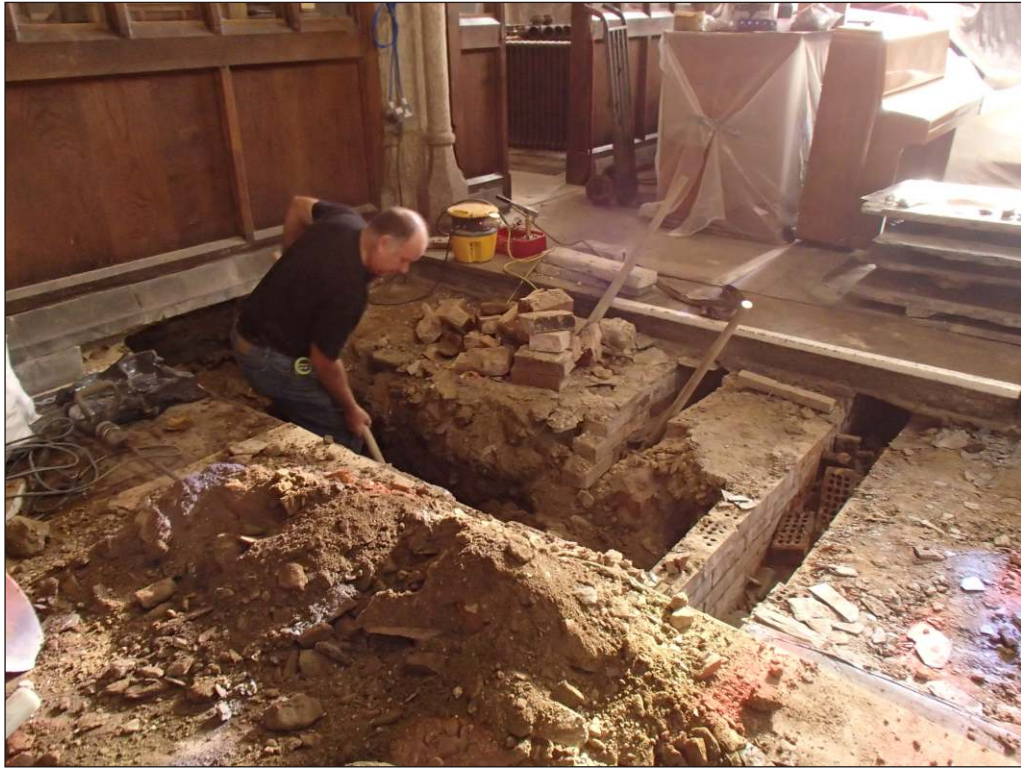
Plate 5: Lady Chapel, works in progress, looking northeast
