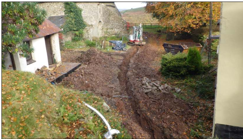
Plate 2. View of cable trench with barn in the background. Looking northeast
