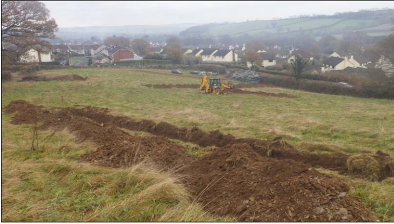
Plate 1: General view of Area 2, looking southeast
