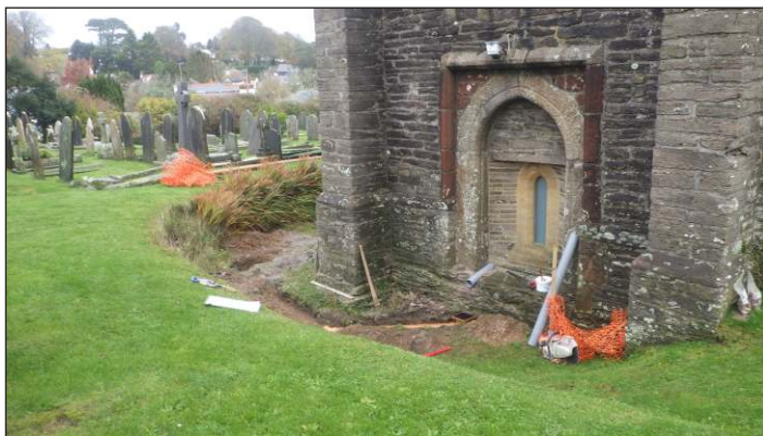
Plate 2: General view of drainage trench. Looking northeast
