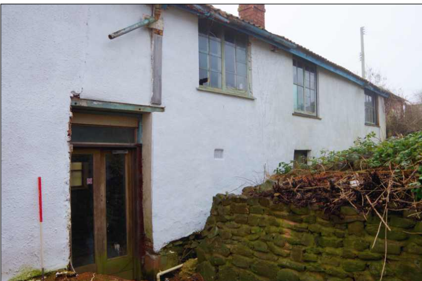
Plate 3: Showing north facing elevation of workshop range. View to southwest (scale 1m)
