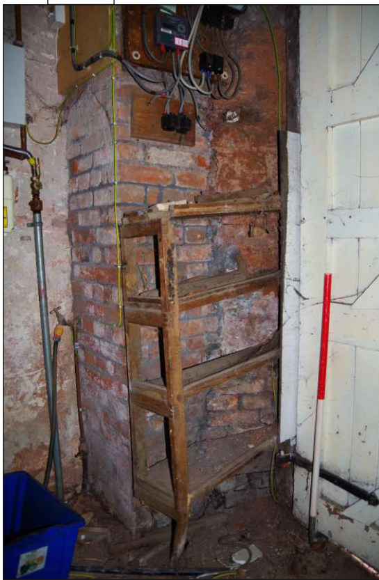
Plate 5: East elevation entrance showing breccia blocks with brick support pillars. View to northeast (scale 1m)
