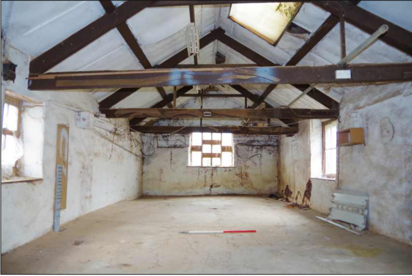
Plate 10: First floor workshop, view to southwest (scale 1m)
