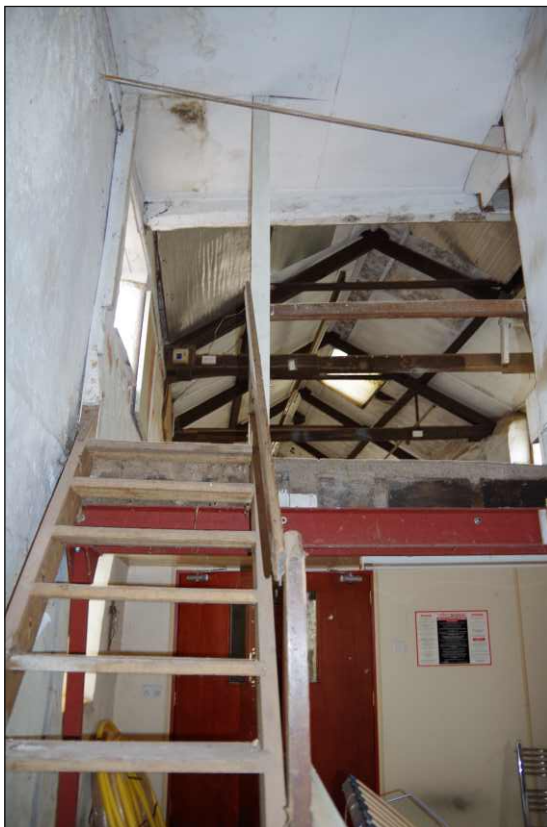
Plate 9: Stairs and first-floor mezzanine area. View to southwest
