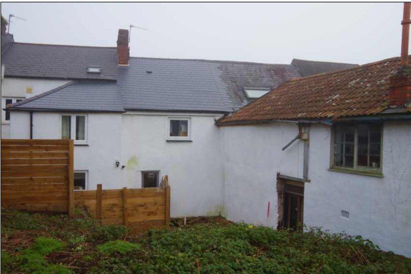
Plate 2: Showing rear of 8 Cockpit Hill with workshop range to the right. View to southeast (scale 1m)
