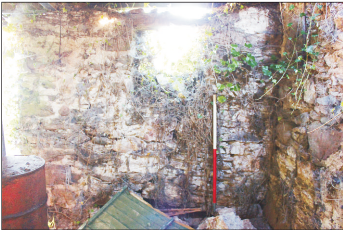
Plate 7: The window in the barn, looking north-northeast. (1m scale)
