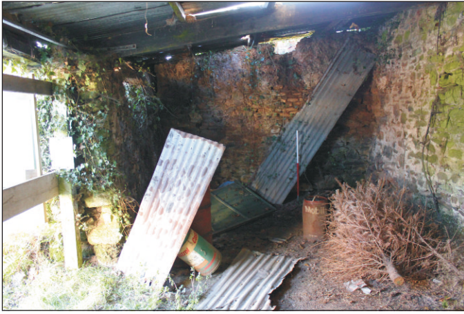
Plate 5: The interior of the barn, looking east-southeast. (1m scale)
