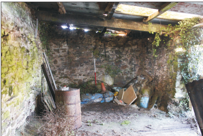
Plate 4: The interior of the barn, looking west-northwest. (1m scale)
