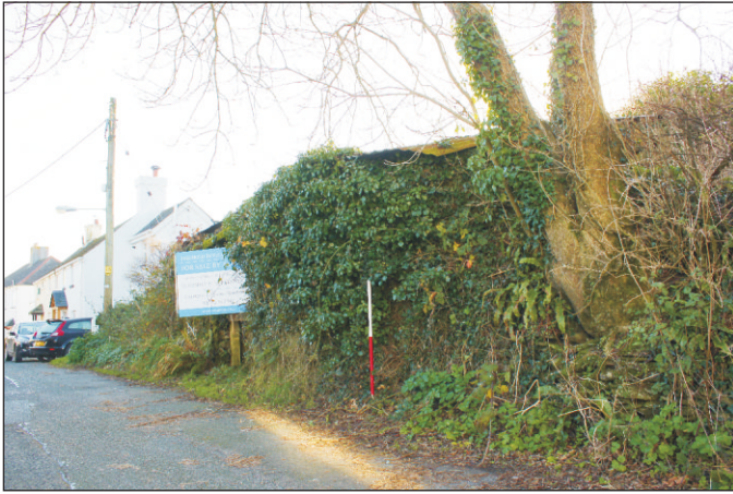
Plate 1: The barn looking southeast along Bovisand Lane. (1m scale)
