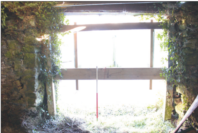
Plate 6: The entrance to the barn, looking north-northeast. (1m scale)
