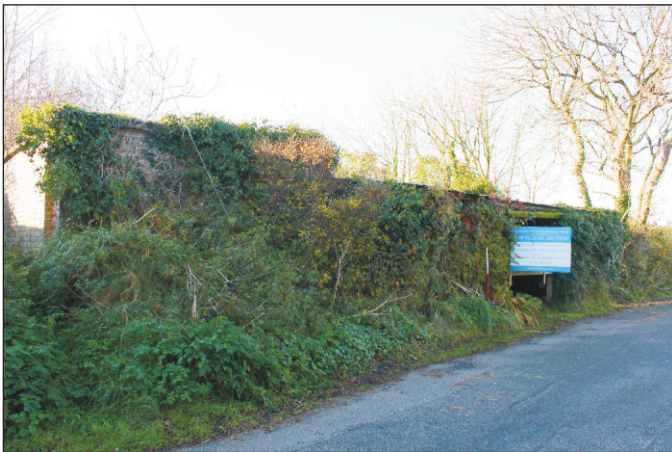
Plate 2: The barn and air raid shelter (foreground) looking west along Bovisand Lane. (1m scale)
