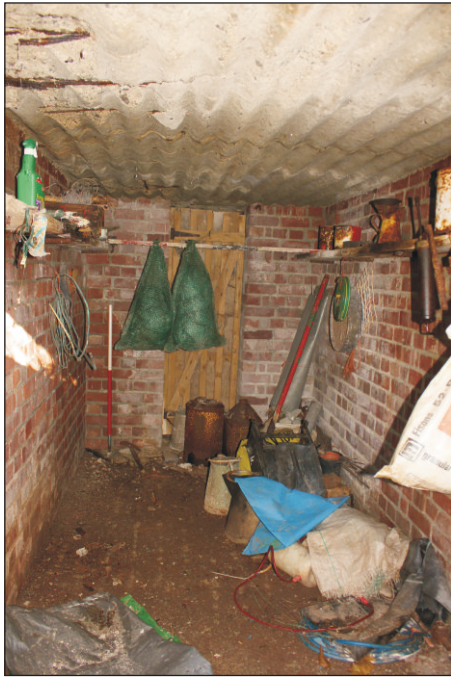
Plate 13: The west room of the shelter, looking north-northeast. (1m scale)
