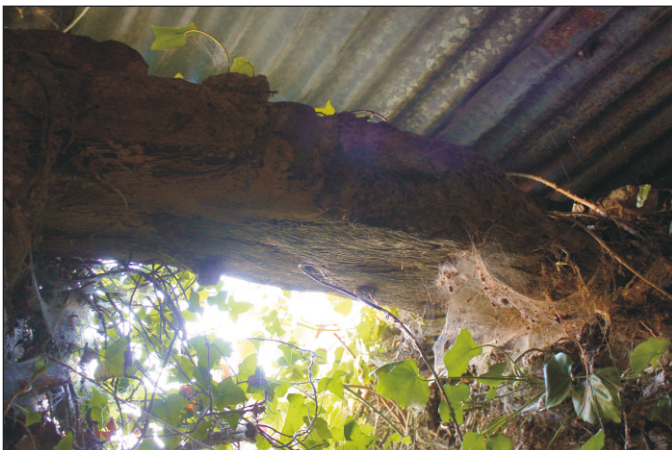
Plate 8: The window lintel showing the pegs, looking northeast
