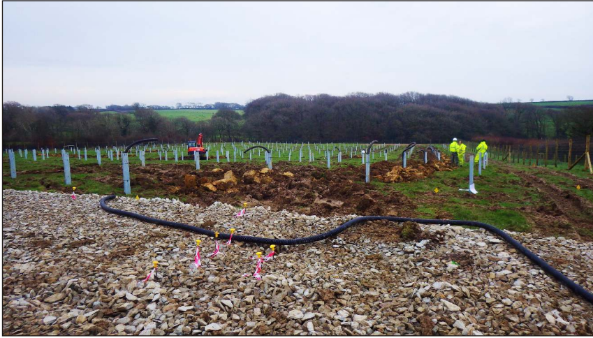
Plate 1: General working view of monitored area looking south-southeast
