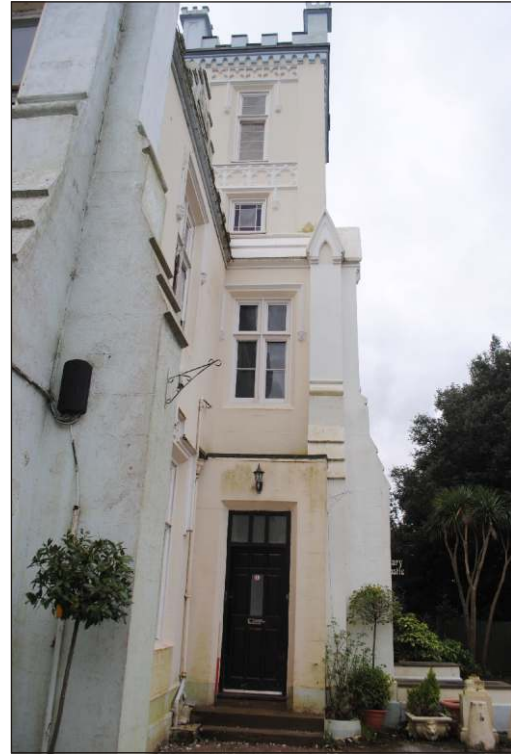
Plate 5: Modern porch added to east side of entrance tower and formerly providing stair access to first-floor apartments, looking west. (1m scale)
