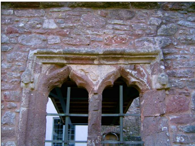
Plate 26: Detail of medieval dripmould with headstops in the early 19th century Brewery Yard wall at Torre Abbey, looking west
