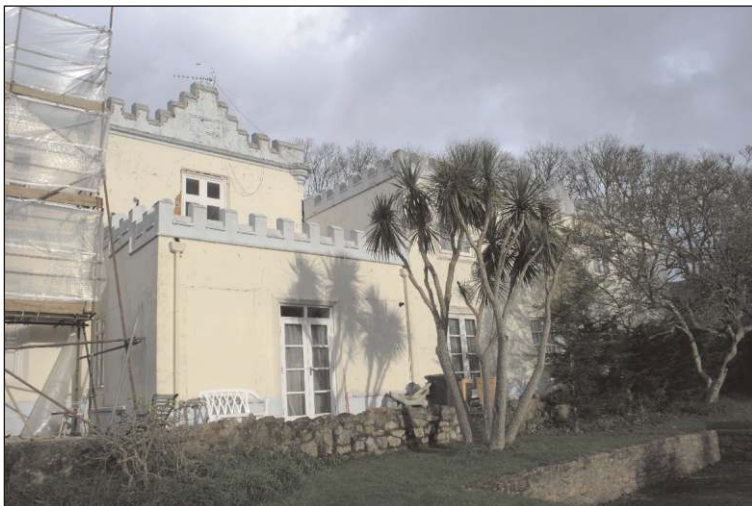
Plate 10: The southeast elevation with primary work with crow step gable visible above the single storey extension, looking northeast
