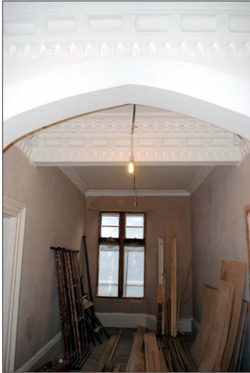
Plate 19: First floor lobby (63) and room (64) viewed from landing (62)
