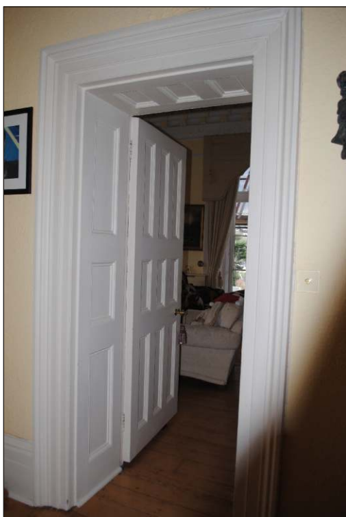
Plate 14: Original internal door between hall (2) and lounge (4)
