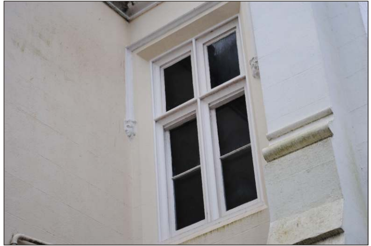
Plate 24: First-floor tower window showing uncomfortable arrangement where the wall junction cuts the dripmould and headstop
