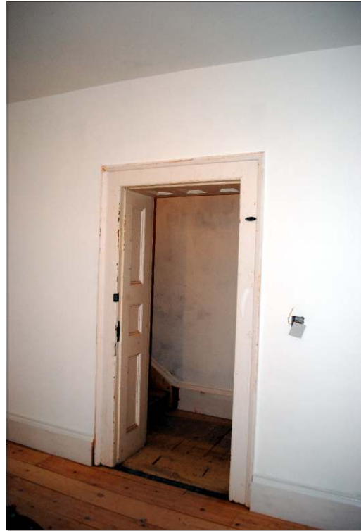
Plate 20: Original doorway in the north wall of room (71), looking northwest
