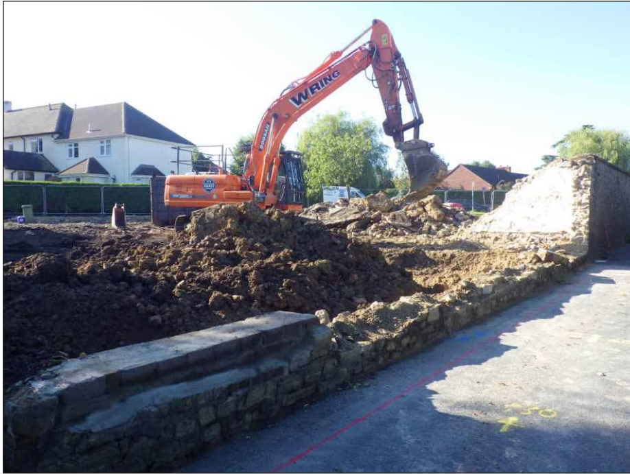
Plate 1: View of site during demolition works. Looking south from Stony Lane
