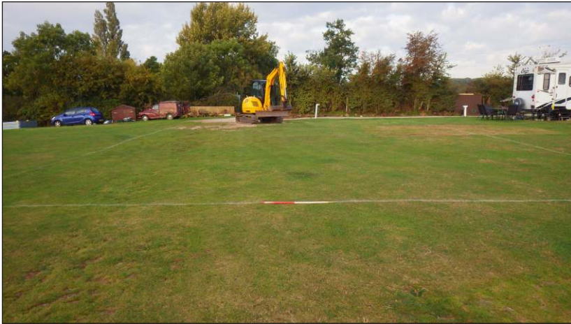
Plate 1: Pre-commencement view of site looking west (scale 1m)
