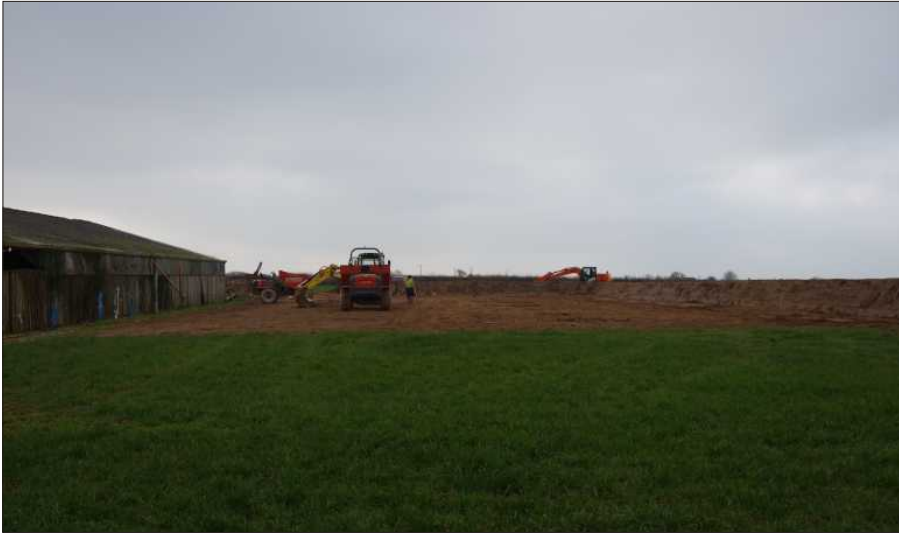
Plate 1: General view of site and area reduced, looking northeast
