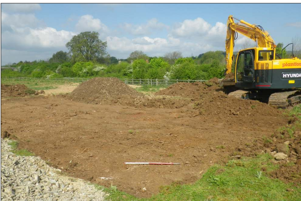
Plate 3: Topsoil stripping, looking northwest. Scale 1m
