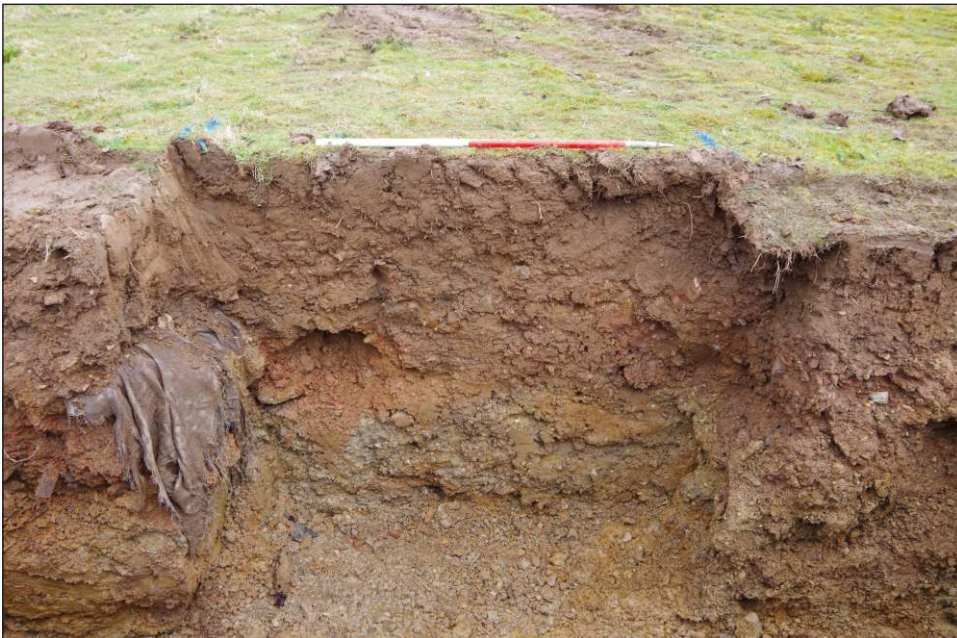
Plate 2: Footing trench, looking east. Scale 1m.
