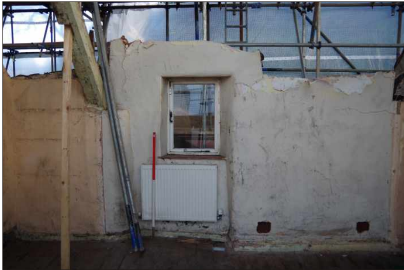
Plate 19: The east side of the north bedroom showing, from left to right, the blocked opening to No. 1 in the north wall, the remains of the north truss, and the window in a possible door opening, looking east. 1m scale.
