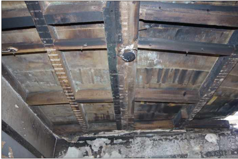
Plate 16: The ceiling of the south bedroom showing the evidence for lath and plaster, with the modern wall lining beyond, looking south
