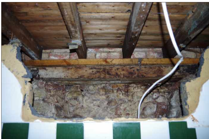
Plate 9: The blocked opening in the south wall of the kitchen, looking south.
