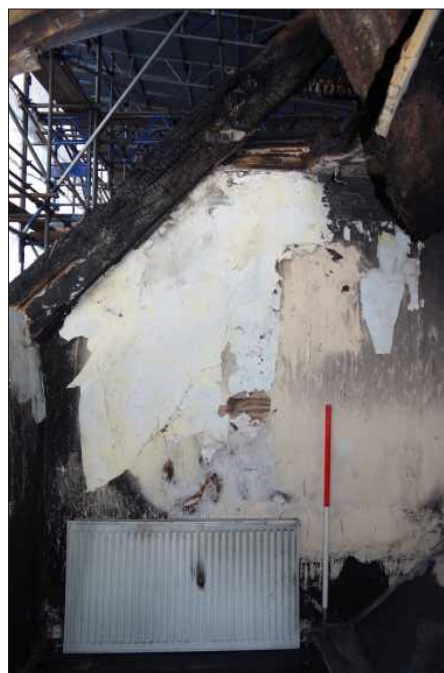
Plate 15: The south bedroom showing the lath and plaster partition with the north bedroom, and part of the enclosed stairs, looking north. 1m scale
