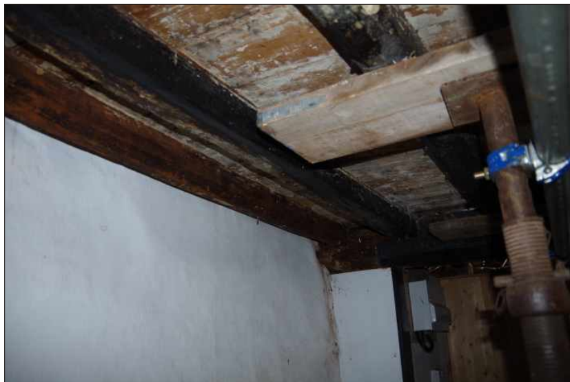
Plate 14: The north end of the bridging beam over the partition showing two of the original joists (to left and right), looking southeast
