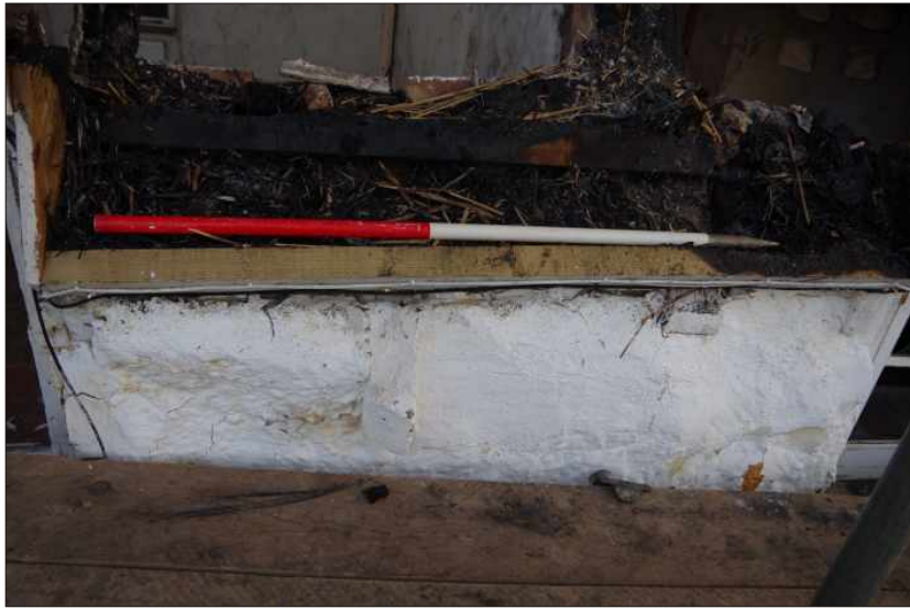
Plate 4: The first-floor masonry of the south elevation showing ends of roof timbers, looking east. 1m scale
