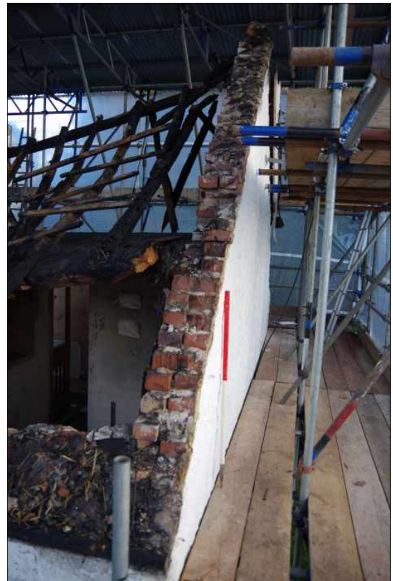
Plate 6: The south gable at first-floor level showing bricks of 20th-century rebuild, looking northeast. 1m scale
