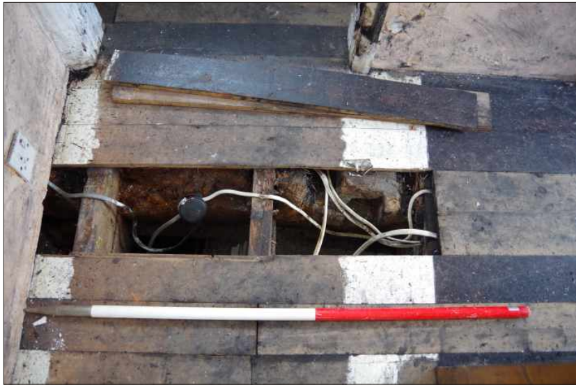
Plate 10: The top of the bridging beam in the kitchen showing former joist sockets, looking south. 1m scale.
