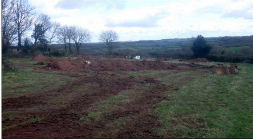
Plate 1: View of the site, work in progress, view from southwest
