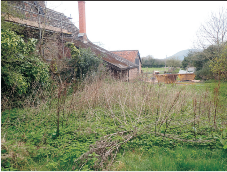
Plate 1: Pre-excitation view of monitored area. Looking north with the site of the Old House to the left
