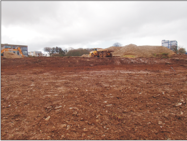
Plate 1: View of the landscaping for the former college with topsoil stripping in the foreground, looking west
