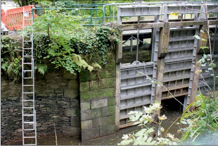
Plate 7: The masonry of and penstocks in the east side of the lock, looking southeast
