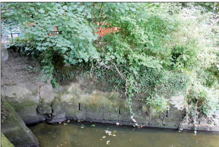
Plate 9: The reused granite masonry in the outflow channel, looking northeast
