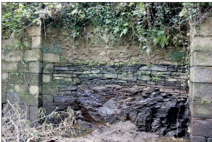
Plate 1: The recess in the west side of the lock showing the bedrock below, looking west
