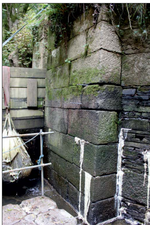
Plate 3: The granite masonry at the north end of the lock showing rebate, looking northeast
