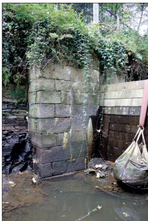
Plate 2: The granite masonry at the north end of the lock showing rebate, looking north
