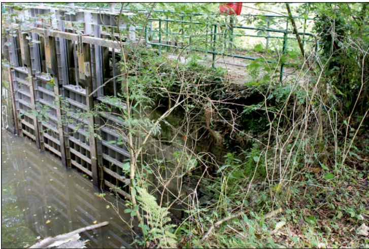
Plate 8: The masonry of and penstocks in the east side of the lock, looking northeast
