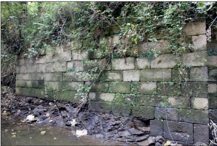
Plate 5: The granite masonry on the west side of the lock showing blocked rebate, looking southwest
