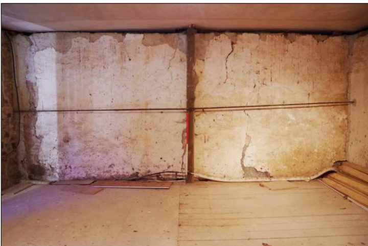
Plate 11: West interior elevation of the hayloft, looking west-southwest. (1m scale)
