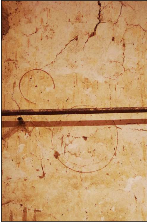
Plate 16: Detail of marks at north end of west elevation, looking west-southwest
