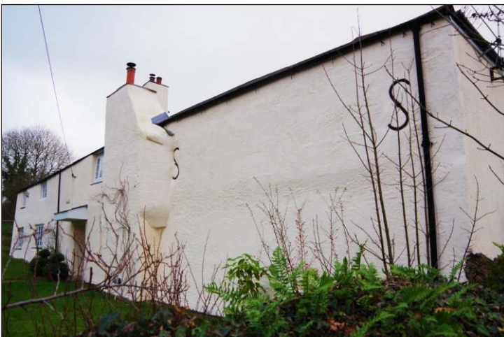
Plate 3: North exterior elevation, looking east
