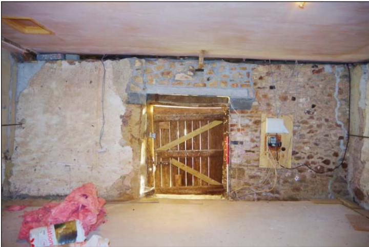
Plate 10: South interior elevation of the hayloft, looking south-southeast. (1m scale)
