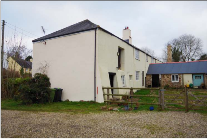
Plate 1: Underhayes viewed from the driveway, looking north. (1m scale)
