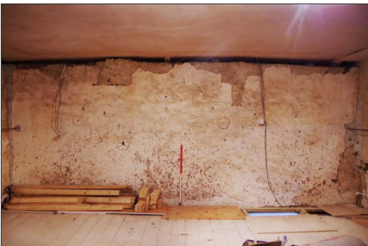
Plate 4: North interior elevation of the hayloft, looking north-northwest. (1m scale)
