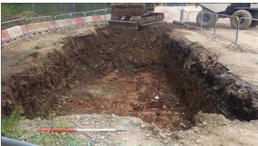
Plate 6: Soakaway tank 1 during excavation, looking southwest. (1m scale)
