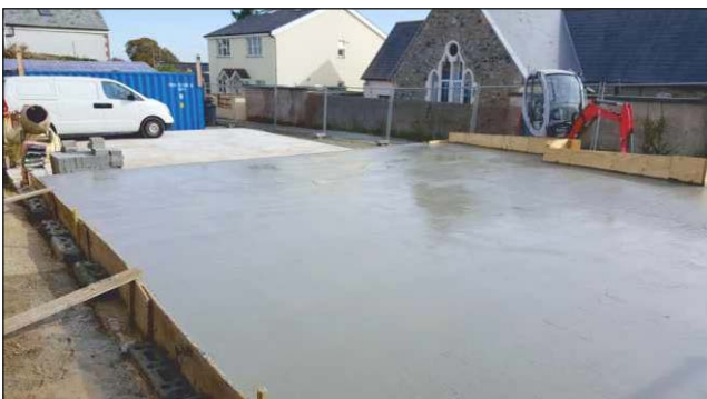
Plate 20: The concrete slab constructed in lieu of foundation trenches, looking southeast
