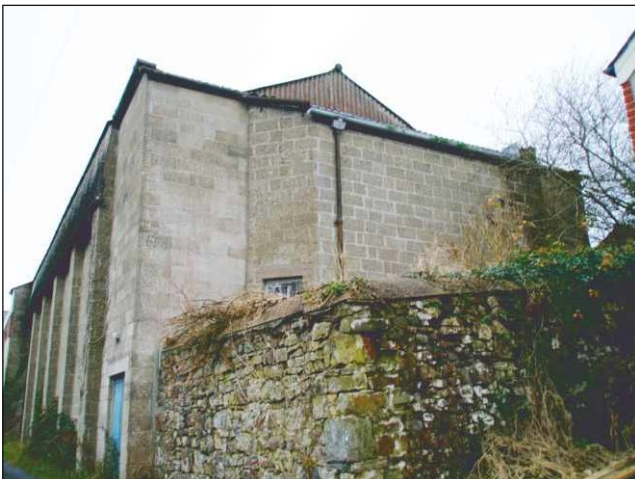
Plate 4: East exterior elevation, looking west
