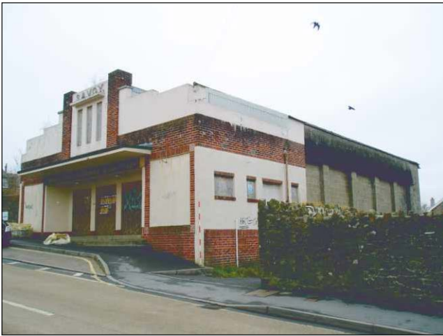
Plate 3: South and west exterior elevations, looking northeast. (2m scale)
