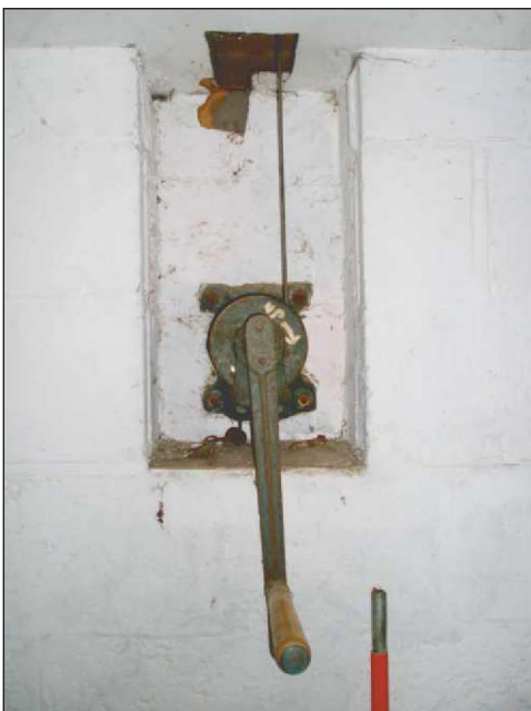
Plate 13: Detail of winding handle in stage area for fly over wires and pulleys
