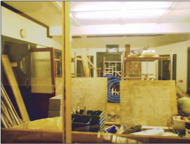
Plate 5: View of foyer, looking north-northwest
