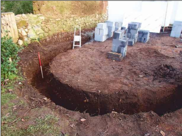
Plate 2: Showing footings trench for new extension. View to east (scale 1m)
