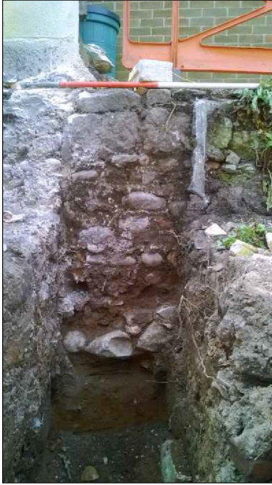
Plate 18: Wall foundations 110 and 109, view from the northeast. 1m scale
