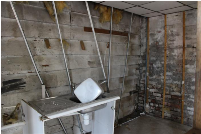
Plate 23: Unit 2, first floor, east corner, looking east
