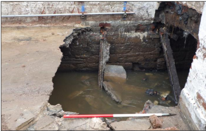
Plate 34: Higher Leat, Zone 6, removal in progress, looking northeast
