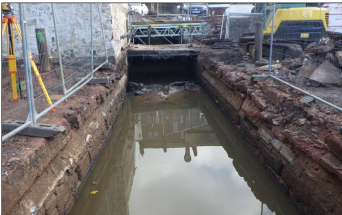
Plate 36: Uncovered Higher Leat, Zones 5 and 6, looking southeast
