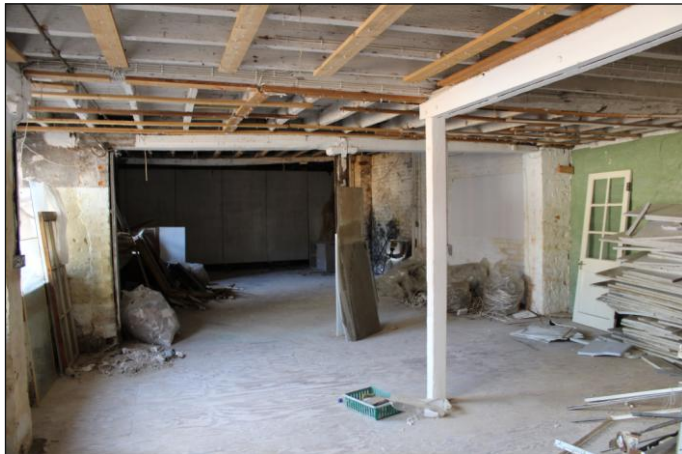
Plate 15: Unit 1, ground floor, general view to northeast end, looking east-northeast
