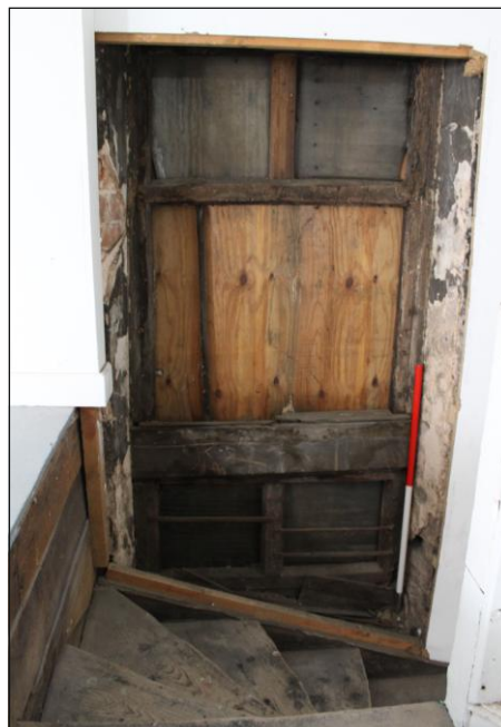
Plate 20: Unit 1, timber frame to window on southeast elevation of the first to second floor stairwell, looking southeast. 1m scale
