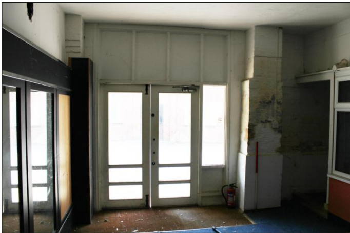
Plate 27: Unit 5, ground floor, southwest elevation, looking southwest. 1m scale
