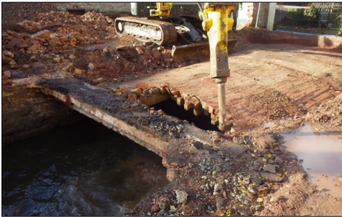
Plate 30: Higher Leat, Zone 2, work in progress, looking west
