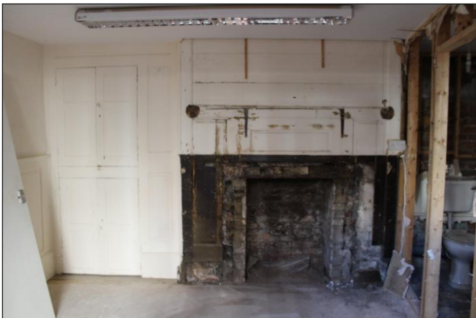
Plate 11: Unit 1A, southeast elevation, looking southeast
