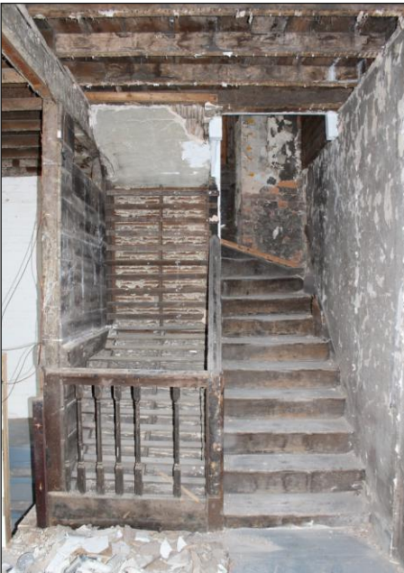
Plate 19: Unit 1, first floor, probable mid to late 18th-century staircase, looking southeast
