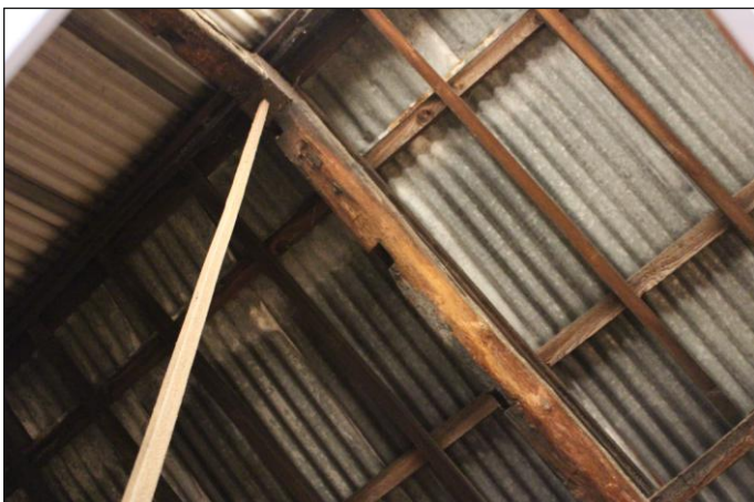
Plate 28: Unit 5, view of A-frame truss and iron king post, looking north
