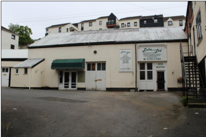
Plate 6: Southwest exterior elevation of the north range, looking northeast
