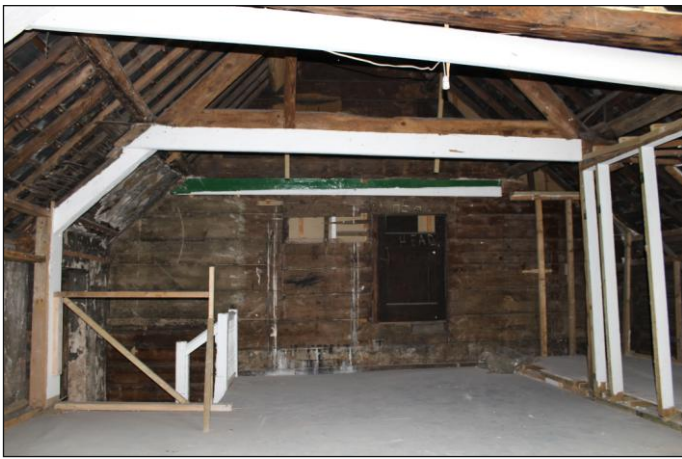
Plate 21: Unit 1, second floor, southwest elevation, looking southwest
