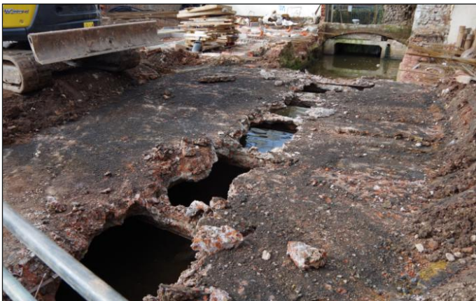
Plate 32: Higher Leat, Zone 4, work in progress, looking west
