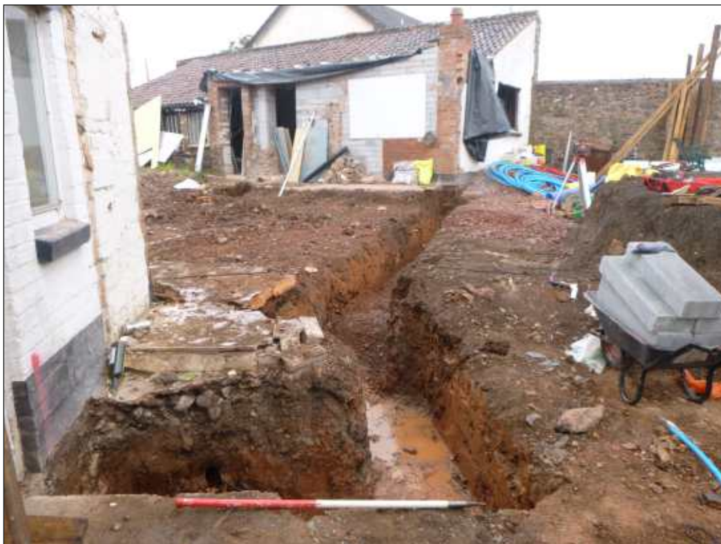
Plate 4: Showing footings trench between Howden Lodge and outbuildings. View to southwest (Scale 1m)
