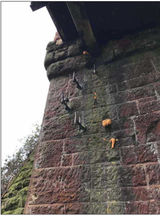
Plate 5: North-facing abutment wall showing cable fittings associated with the former railway
