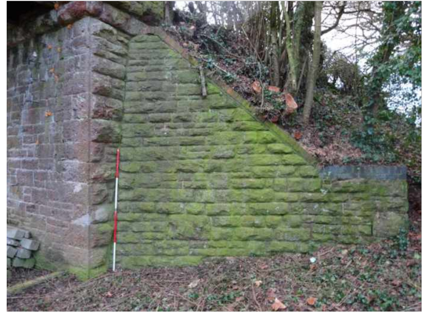
Plate 6: North-facing elevation of south wall abutment (scale 2m)
