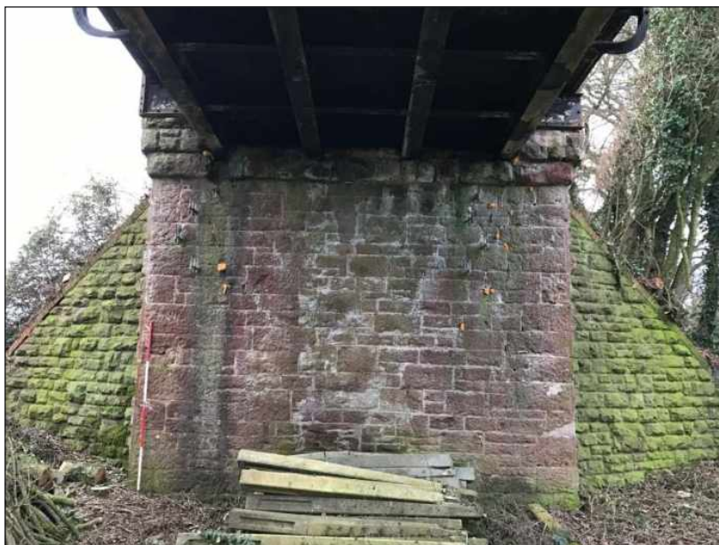
Plate 3: North-facing elevation of abutment wall (scale 2m)
