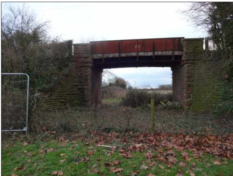
Plate 1: West-facing elevation of bridge (scale 2m)
