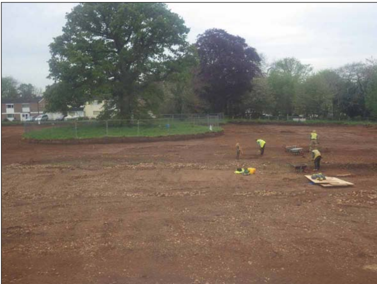
Plate 2: General view of excavation area 3, work in progress, looking south, with area 1 in the foreground
