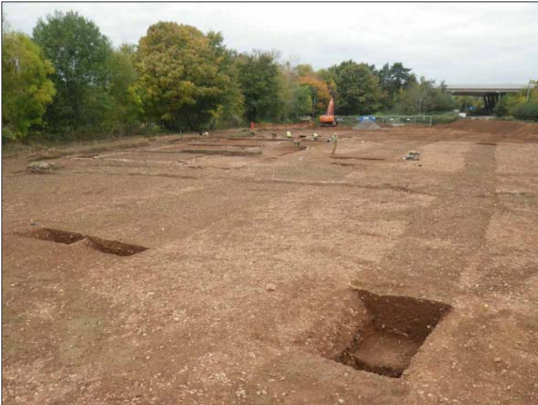
Plate 1: General view of excavation area 1, work in progress, looking southwest
