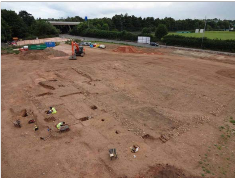
Plate 8: Romano-British building (Structure 3), work in progress, looking northwest
