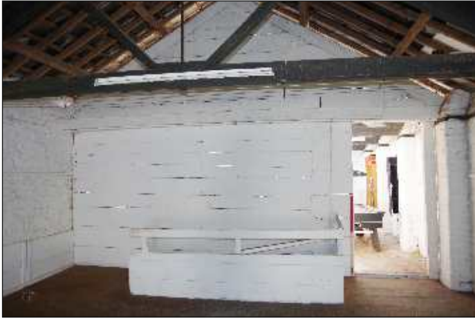
Plate 25: The first-floor partition wall, looking southeast. 1m scale
