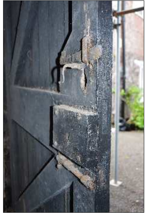
Plate 14: Detail of latch and lock case of the door leading to the exterior from the cider press room, looking south-southeast
