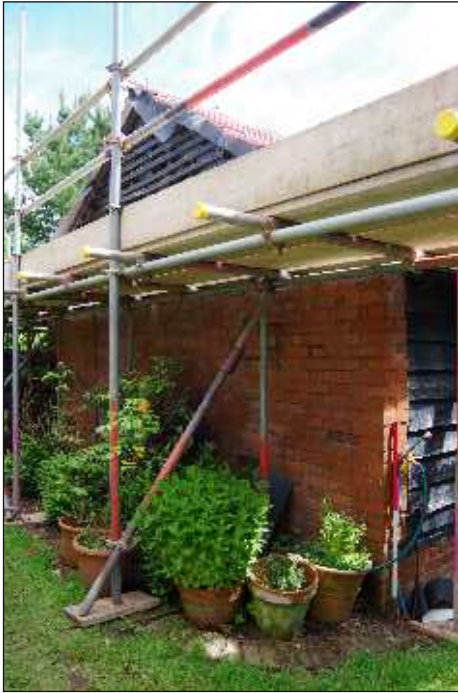
Plate 9: Northwest elevation of chicken coop, looking northeast. 1m scale
