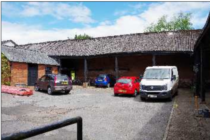
Plate 2: General view of the north range of the linhay, looking northeast
