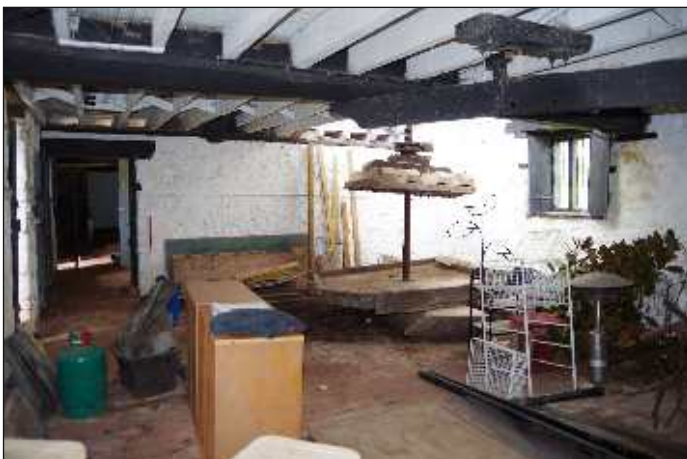
Plate 12: General view to the northwest end of the cider press room, looking northwest. 1m scale
