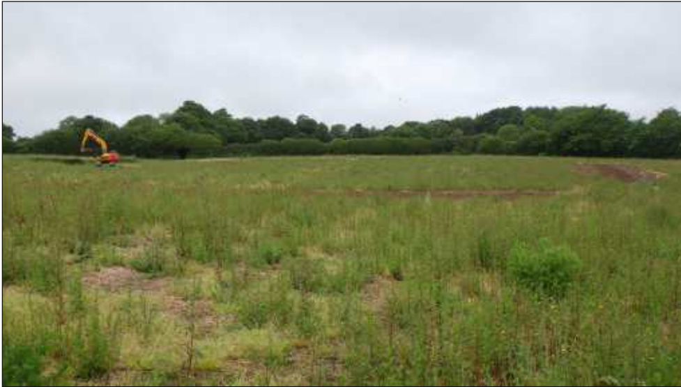
Plate 1: View of the site, work in progress, looking to west
