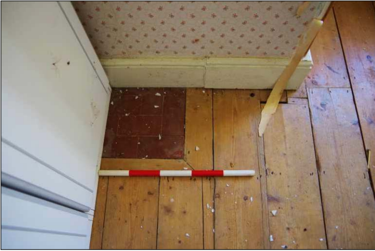
Plate 21: Room 8, detail of fireplace tiles and replaced skirting, looking south-southwest. (0.5m scale)
