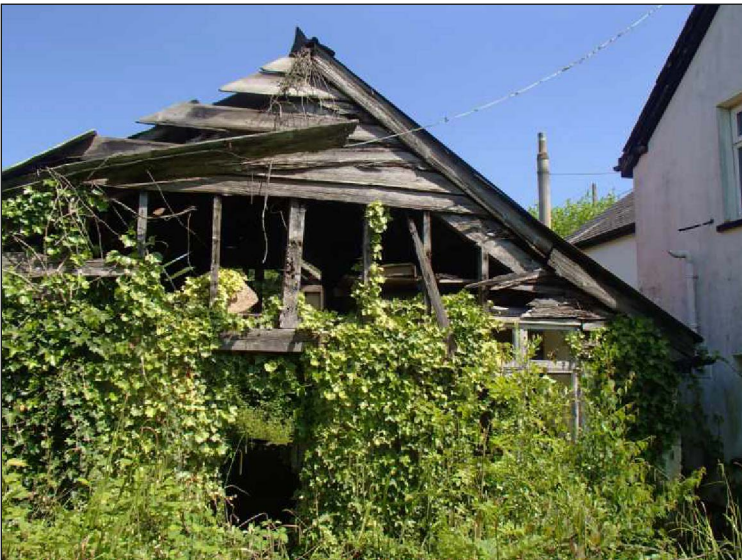
Plate 23: South elevation of outbuilding, looking north-northeast
