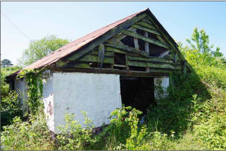
Plate 22: North and east elevation of the outbuilding, looking south
