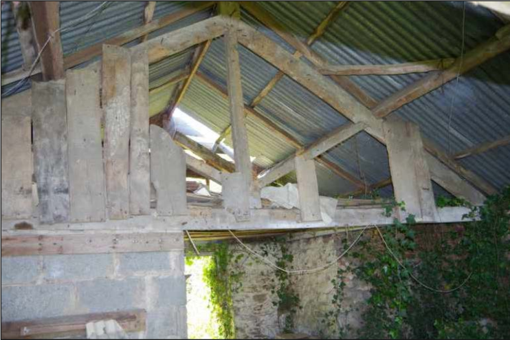
Plate 24: View of interior of outbuilding, showing central A-frame truss, looking southwest
