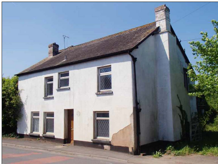
Plate 7: North gable end and east elevation of Stoke Cottage, looking west-southwest
