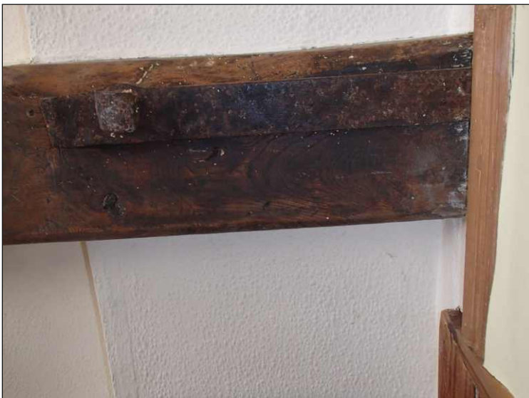
Plate 12: Room 1, detail of iron strap and bolt fitting to beam at west end, looking south-southwest
