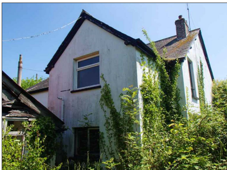
Plate 9: South end of west elevation of Stoke Cottage, looking east
