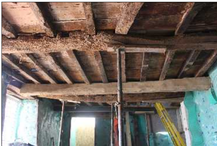
Plate 7: Part of the first-floor structure, looking south.
