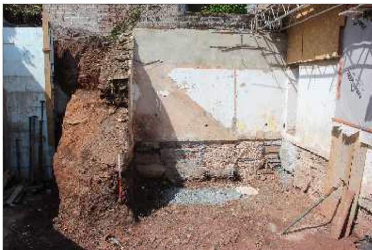
Plate 16: The extension showing remains of south wall, looking west. 1m scale
