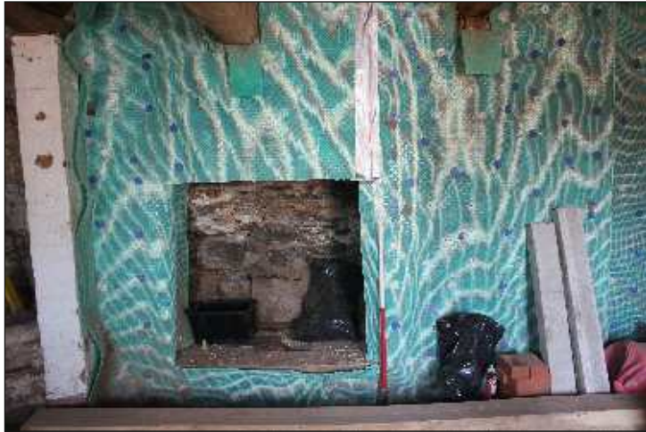
Plate 5: The ground-floor fireplace, looking west. 1m scale
