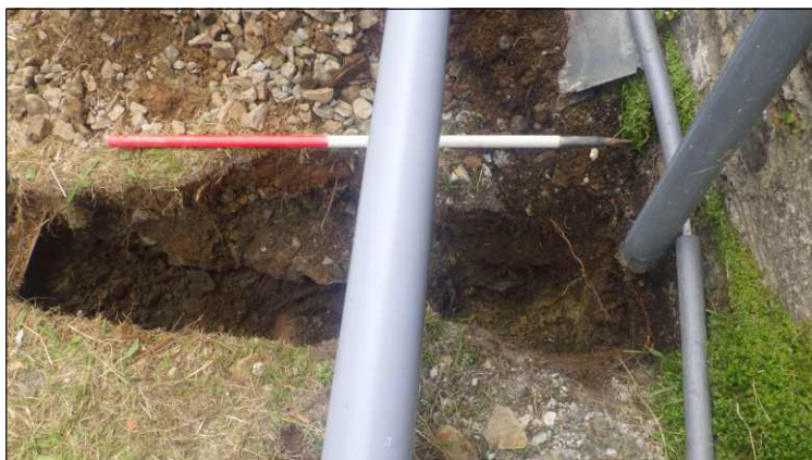
Plate 3: Showing detailed view of new drain connection trench. View to south (scale 1m)
