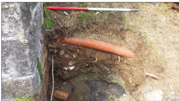
Plate 4. Showing pit for new inspection chamber. View to west (scale 1m)
