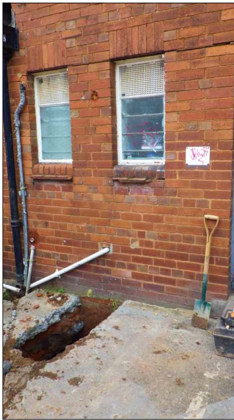
Plate 11: Location of test pit 6, looking southwest
