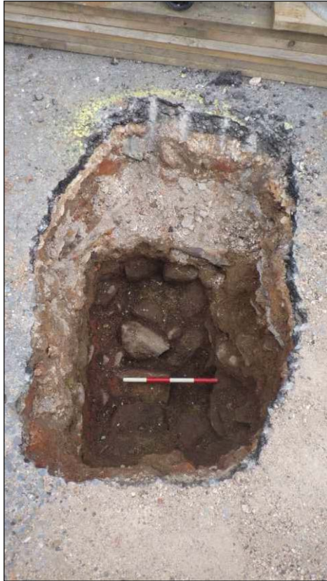
Plate 8: View of test pit 4, showing loosely-bonded volcanic trap wall 408. Looking northeast. (Scale 0.4m)
