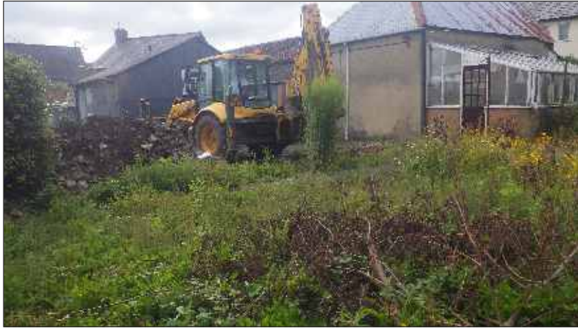
Plate 1: General site view. Looking southeast
