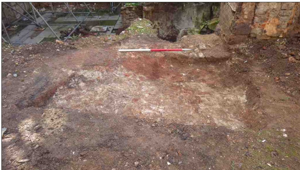
Appendix Plate 6: The investigations looking southwest. 1m scale
