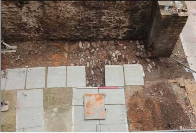
Plate 9: Test pit 5, cobbled surface 505 looking northwest down from the scaffolding over the cellar. (1m scale)
