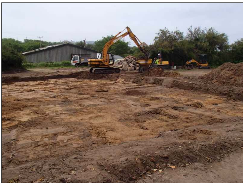
Plate 1: General view of site, work in progress, looking southwest
