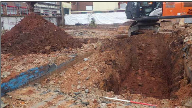
Plate 3: Trench 3, work in progress, looking northwest (1m scale)
