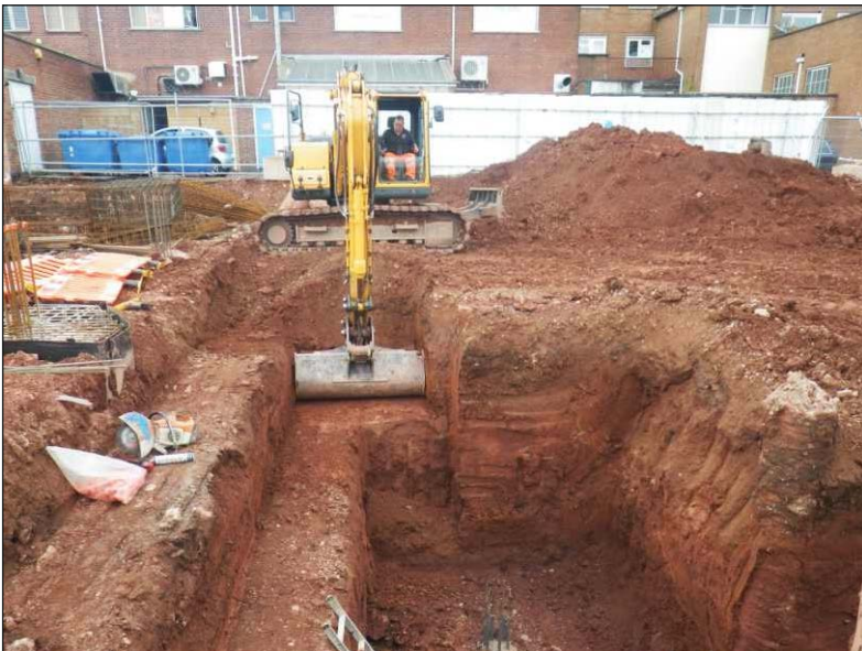
Plate 2: Watching brief area, basement groundworks, work in progress, looking northwest
