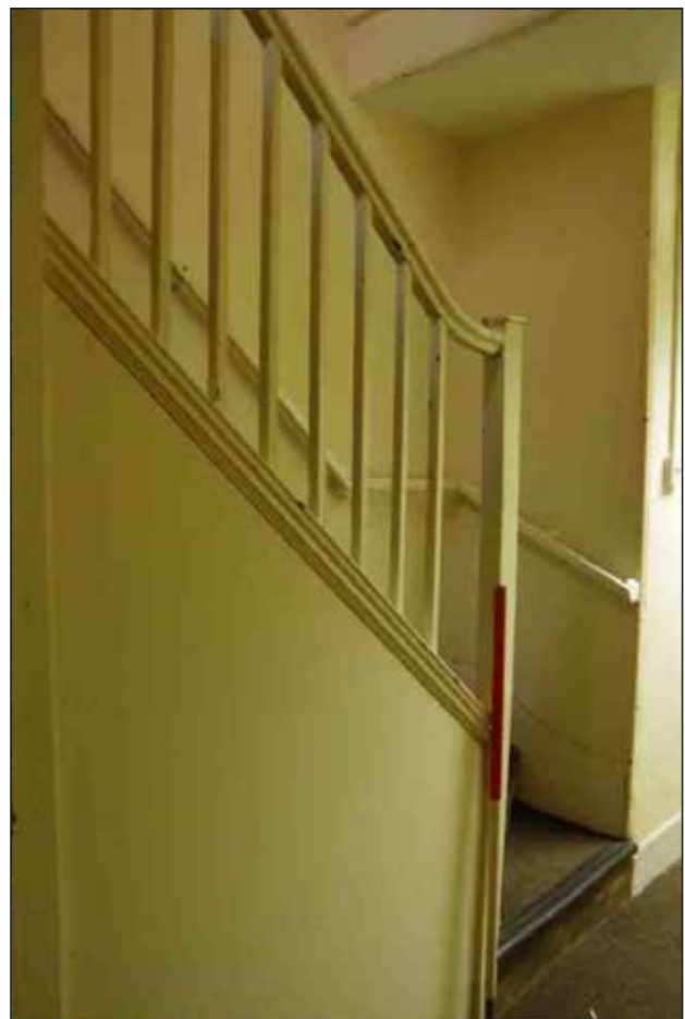
Plate 27: Staircase in rear range of the house, looking southeast (1m scale)
