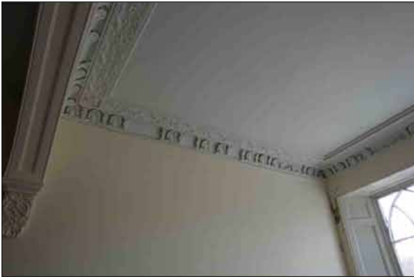
Plate 17: The ceiling of the stairwell on the first floor, looking northwest
