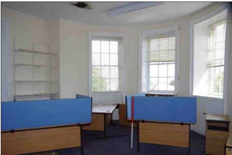
Plate 23: General view of southeast room on the first floor, looking southeast (1m scale)
