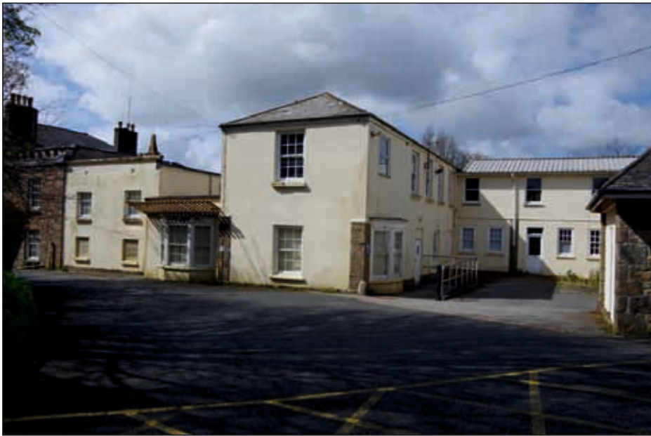
Plate 37: General view of original stable block, infill buildings and later stable block, looking southwest
