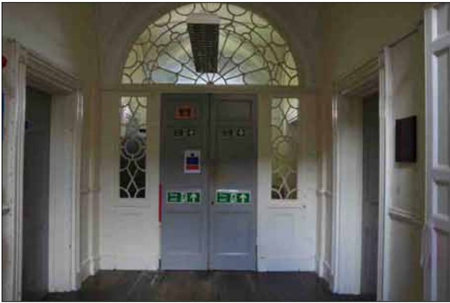
Plate 7: Wooden doors with decorative tracery dividing the reception areas looking southeast (1m scale)
