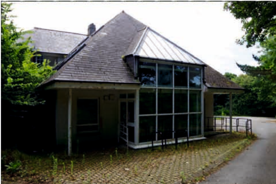
Plate 60: Northwest elevation of the extension, looking south
