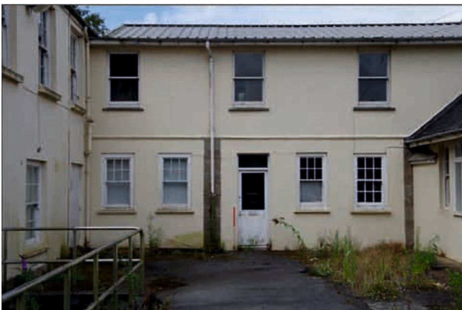
Plate 46: Northeast elevation of later stable block, looking southwest (1m scale)
