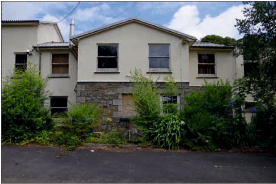
Plate 47: Southwest elevation of later stable block, looking northeast (1m scale)
