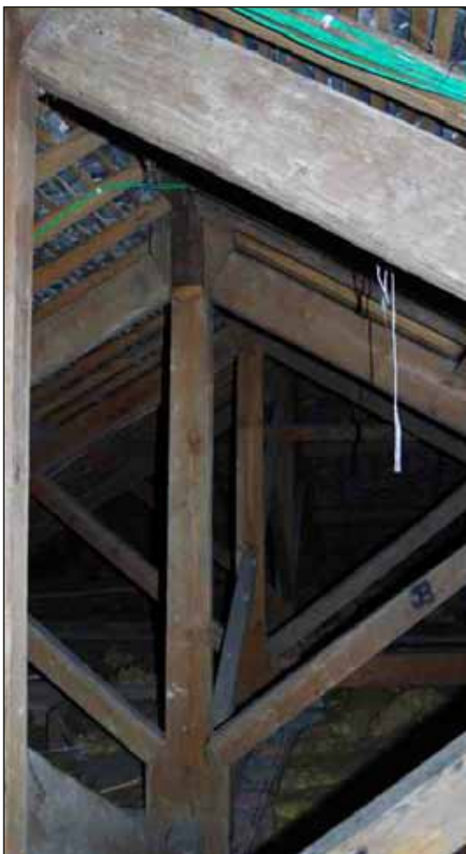
Plate 26: King post roof trusses, looking southwest
