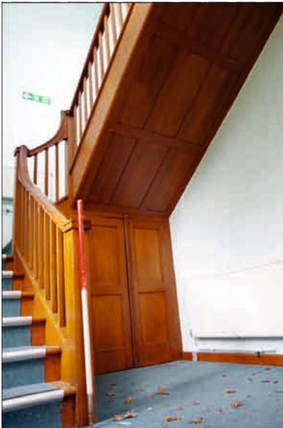
Plate 55: Stairs in the dining hall building, looking northwest (1m scale)
