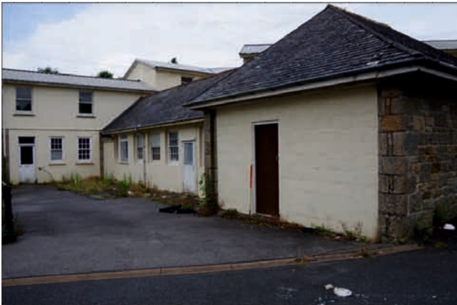
Plate 45: Southeast elevation of later stable block, looking northwest (1m scale)
