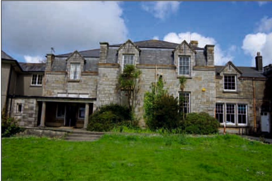
Plate 50: Southeast elevation of the dining hall building, looking northwest
