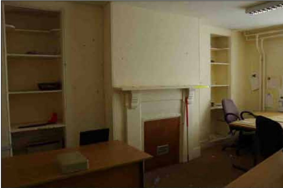
Plate 28: General view of southwest room on the ground floor of the rear range, looking southwest (1m scale)
