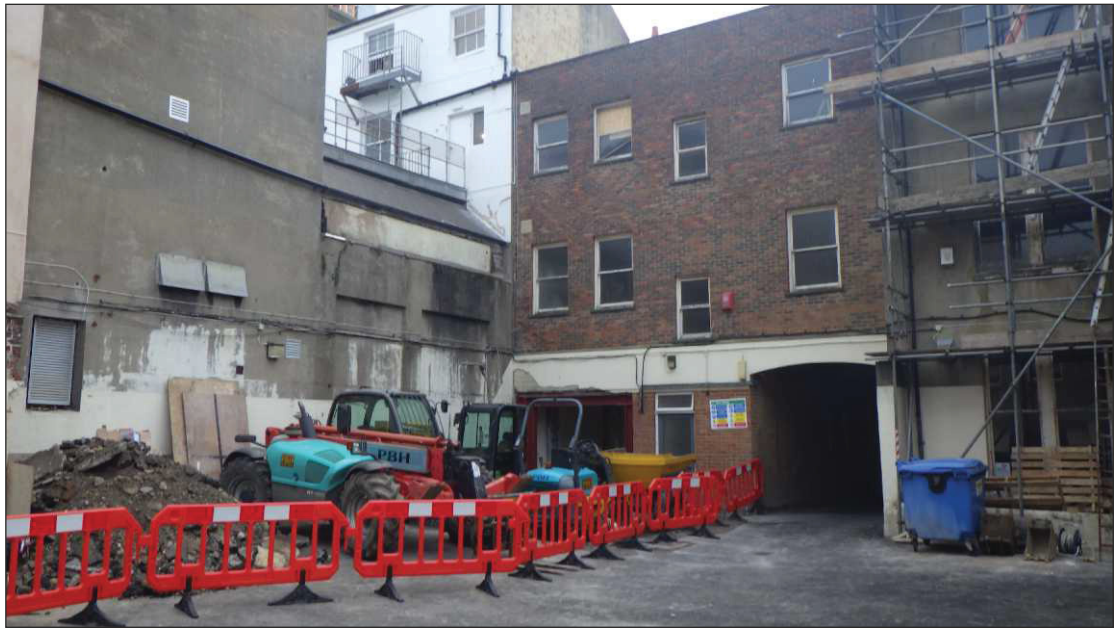
Plate 1: General view of site, looking northeast
