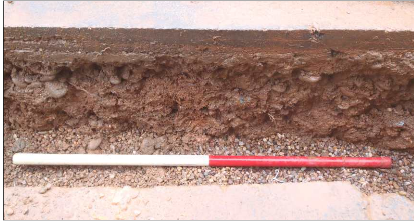
Plate 4: Representative section in the northwest end of the drainage trench, looking southwest (1m scale)
