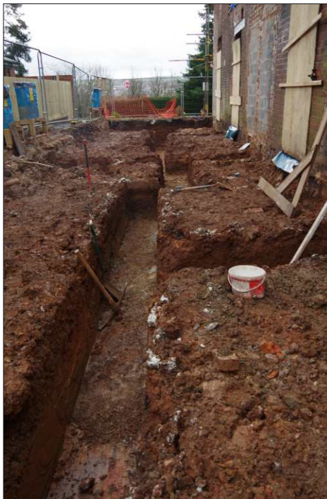
Plate 8: General view of foundation trenches in block E, looking southwest
